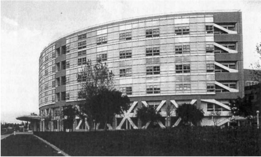
Figure 13.6 Arrowhead Regional Medical Center. (Courtesy of KPFF Consulting Engineers.)
