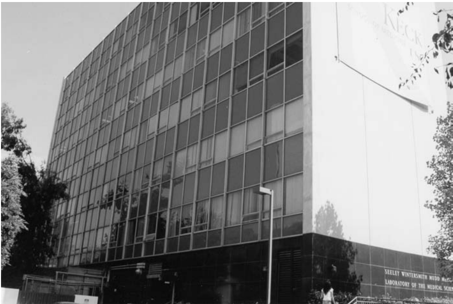
Figure 1.10 It is estimated that 80% of hospital structures in California are of the moment frame–shear wall type of construction, a bad design arrangement to resist a strong earthquake.
