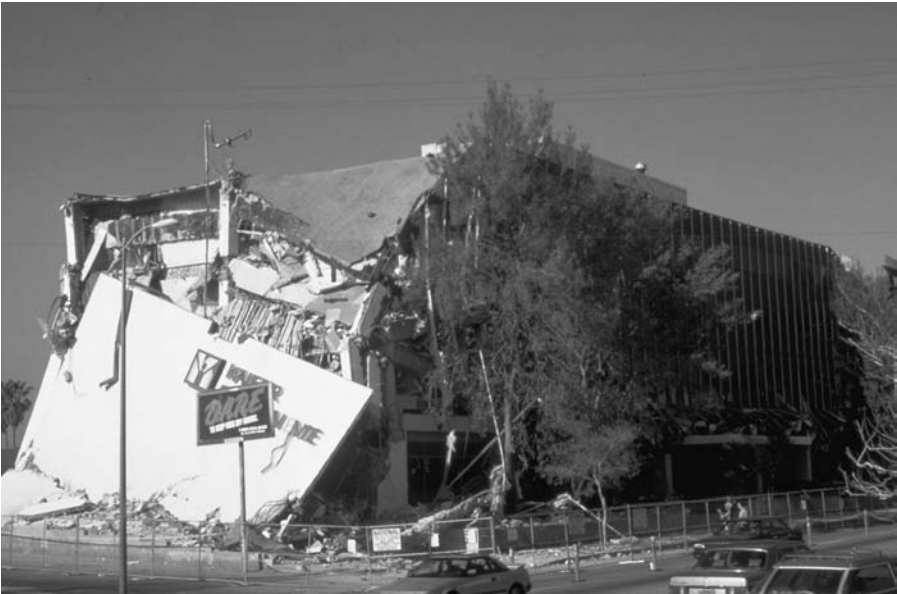
Figure 1.7 Northridge earthquake, 1994. Collapsed end shear wall, Kaiser Permanente Office Building, Granada Hills, CA. (Photo courtesy of the University of California Library at Berkeley.)
