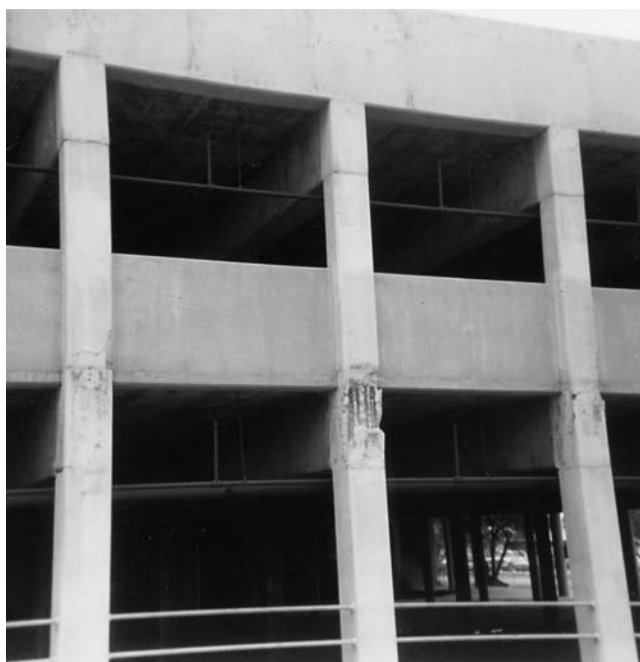
Figure 1.18 Initial stages of column joint degradation in the progressive failure of a fashion center parking structure in the Whittier Narrows earthquake, 1987.
