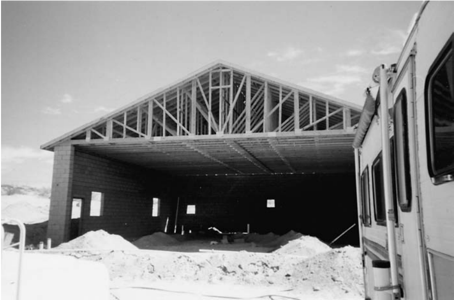
Figure 7.5 Partial view of the hangar during construction.
