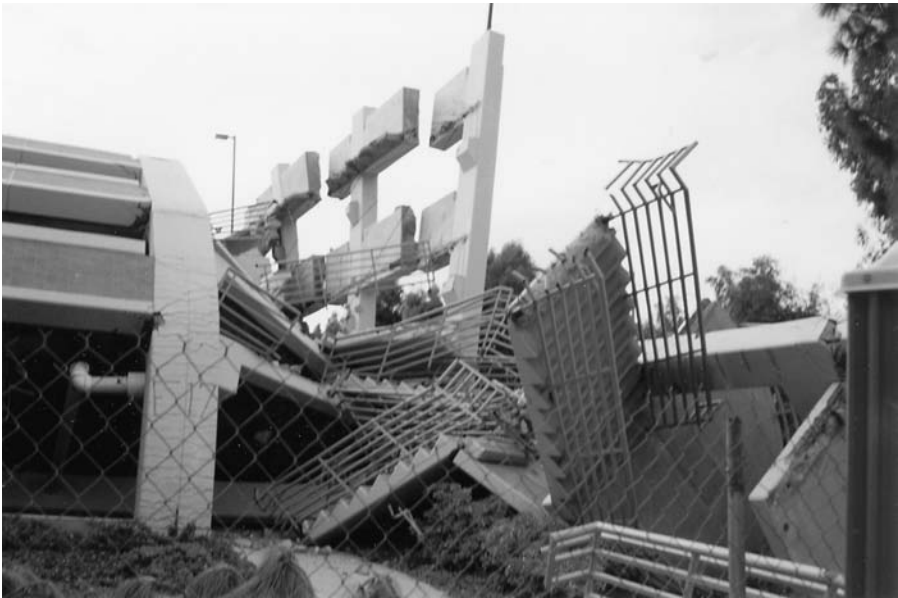
Figure 1.14 California State University parking structure. A corner of the cast-in-place framework was pulled in by the collapsed interior of the multistory structure during the 1994 Northridge earthquake.
