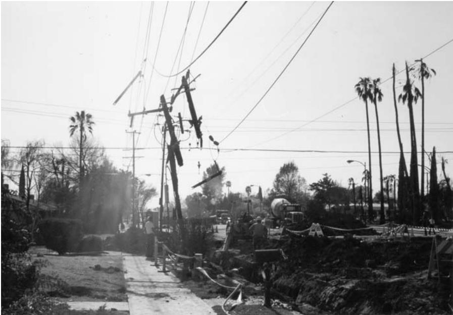
Figure 12.1 Overall damage on Balboa Boulevard near the epicenter of the Northridge earthquake.
