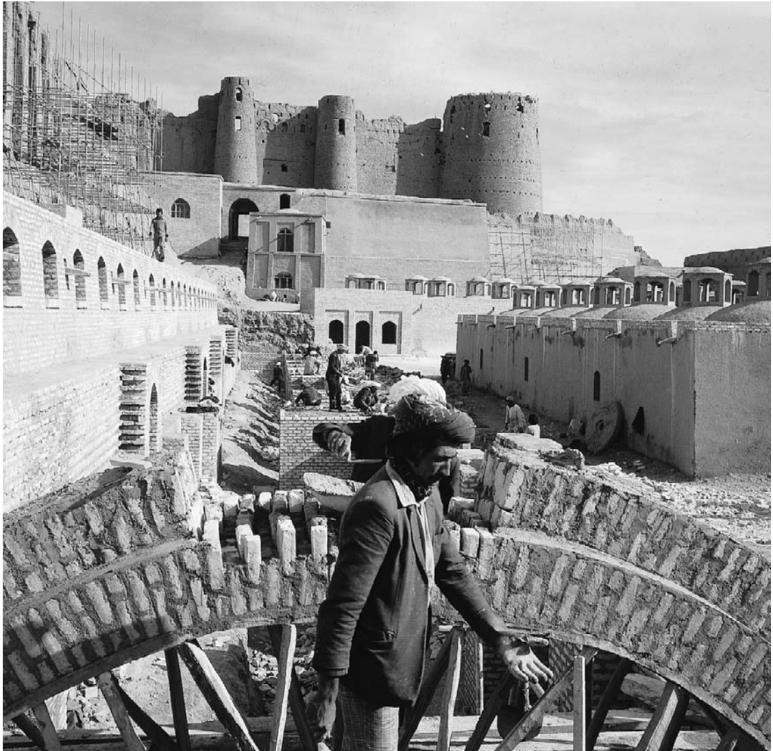
Figure 10.18 The use of traditional technology in the restoration of ancient vaults at Herat in Afghanistan challenges the interpretation of modern restoration concepts in a traditional context. UNESCO project in 1974–80. (A. Bruno)
