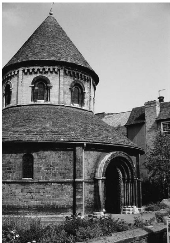
Figure 6.19 The Round Church of Cambridge was restored by A. Salvin around 1845, reflecting the guidelines of the Ecclesiological Society. The conical roof replaced an earlier embattled tower
