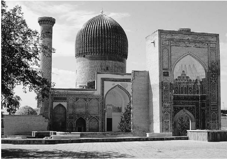
Figure 10.7 The main portal and ribbed dome of Gur-i Amir mosque (1404) in Samarkand were restored on the occasion of Timur's Jubilee in 1996. Like this mosque, which contains Timur's tomb, many of the historic monuments of Samarkand have been isolated from the urban fabric that used to surround them
