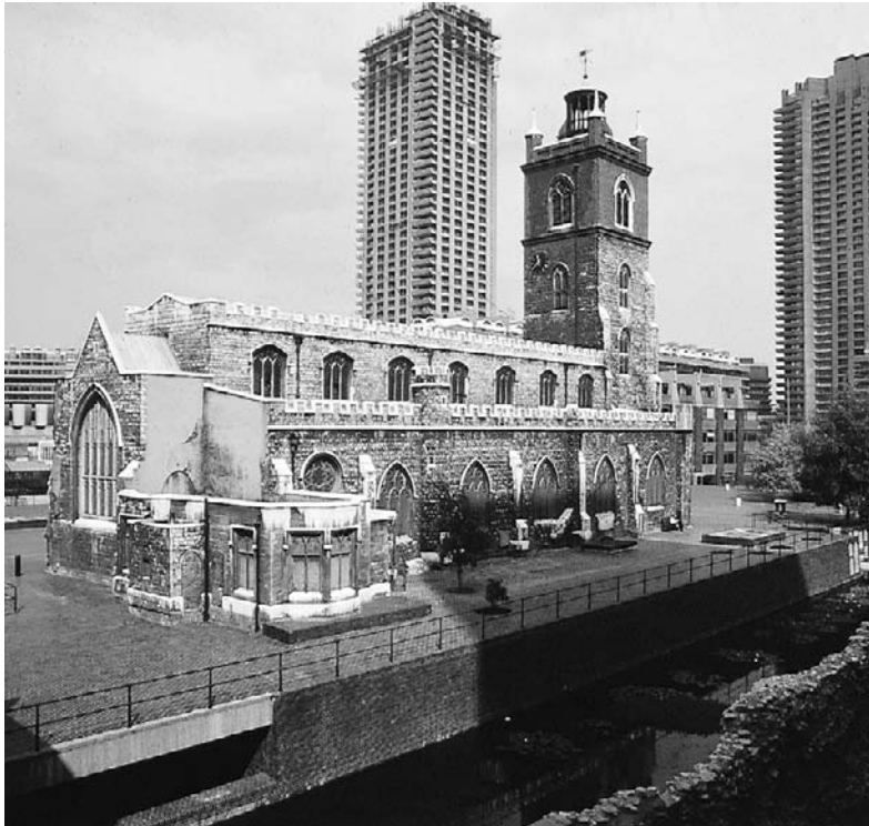
Figure 8.13 Insensitive planning can destroy the relationship of a historic building with its context. This example from the Barbican area, London
