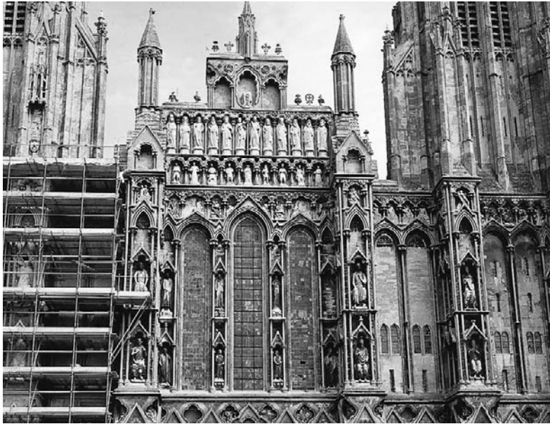
Figure 8.11 The front of Wells Cathedral was conceived and built together with the statues; its potential unity is expressed in all its elements. Any interventions, such as cleaning or consolidation, should be carried out with clear understanding of this relationship. Removal of the statues from their context would damage the architectural, historical whole of the cathedral
