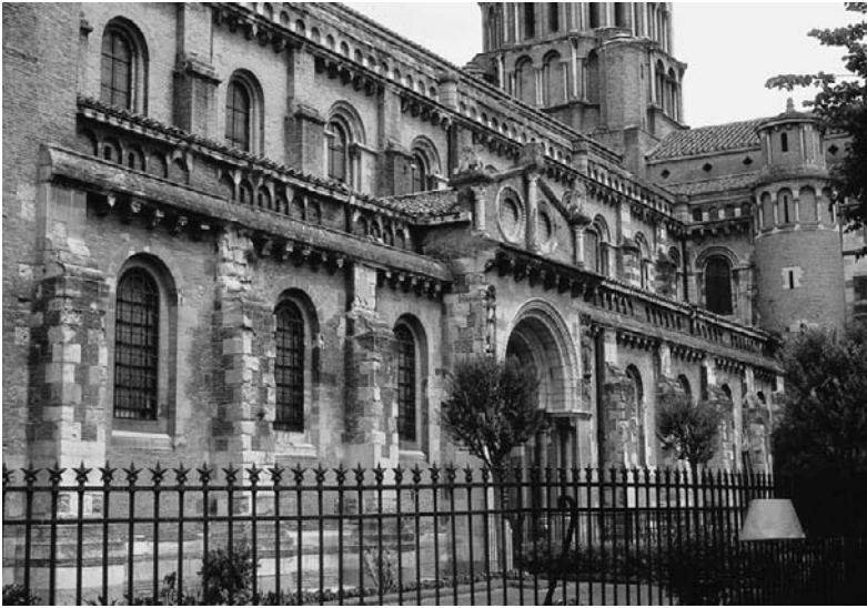
Figure 6.15 The church of Saint-Sernin in Toulouse was reinstated by Viollet-le-Duc to the 'condition of completeness' represented by its Romanesque style. This meant removal of later, Gothic modifications. The first plans were prepared in 1847, based on archaeological examination, and the works initiated in 1860
