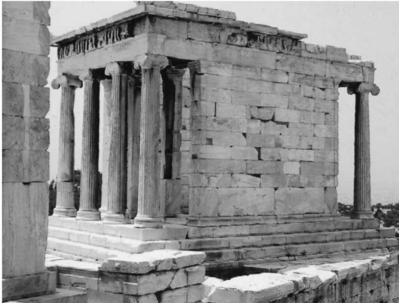
Figure 7.6 Temple of Nike in Athens after the second restoration in the 1930s
