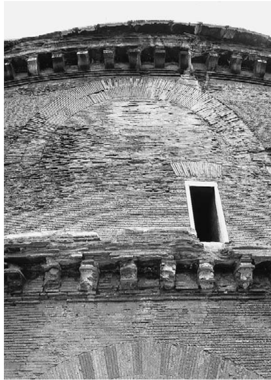
Figure 8.18 Reintegration of old, weathered and consumed surfaces demands sensitivity so as not to emphasize the visibility of new parts at the cost of reducing the originals. An example of reintegration in the brick wall of the Pantheon, Rome
