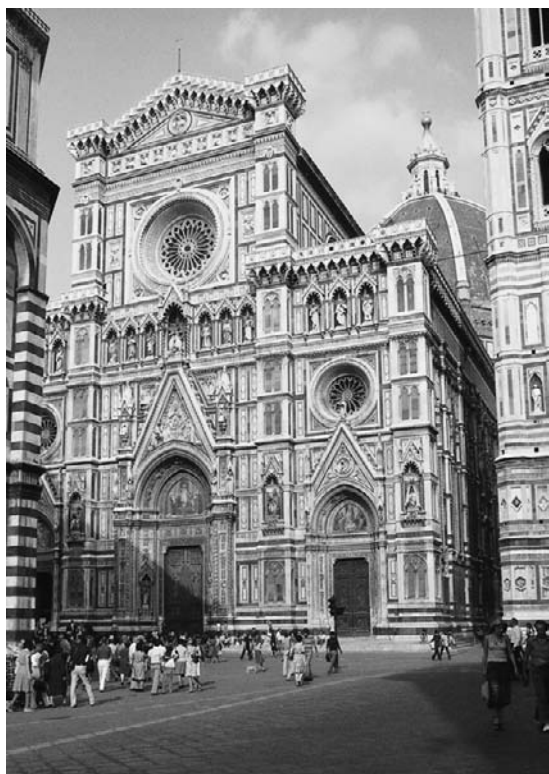
Figure 6.25 The principal elevation of Florence Cathedral was built to the design of Emilio de Fabris, who won the competition in 1868
