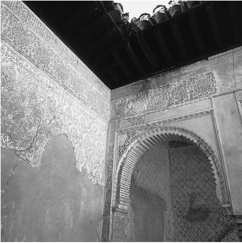
Figure 9.5 La Alhambra, Palacio de los Leones, Patio del Harén . Detail of the west portico in which are visible the criteria used by L. Torres Balbás in the 1920s. The work consisted of the reconstruction of the original space and the general decorative frame. The block of the reproduced element is left without decoration. ( Consejo Superior de Investigaciones Científicas )
