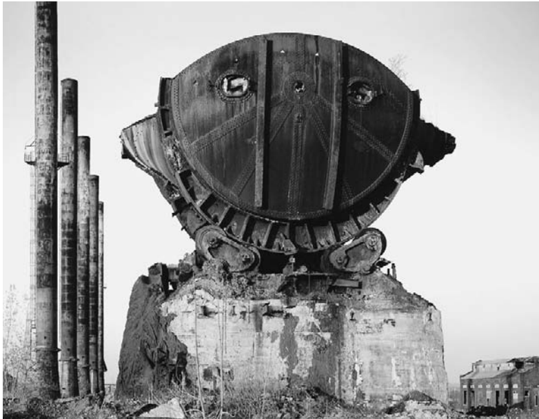
Figure 9.26 The Mixer Ruins in Ensley, Birmingham, Alabama, are an example of protected industrial heritage in the USA. The site belonged to Tennessee Coal and Iron Company and was active from 1899 to 1980. (Photo: Jett Lowe. HABS/HAER Collection, Prints and Photographs Division, Library of Congress)
