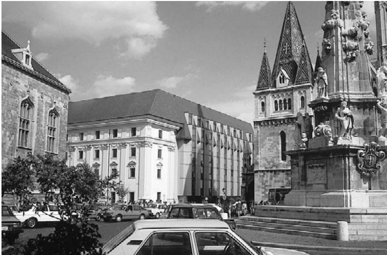
Figure 9.21 The relatively large modern complex of the Hilton hotel was integrated within historic structures in the Old Buda
