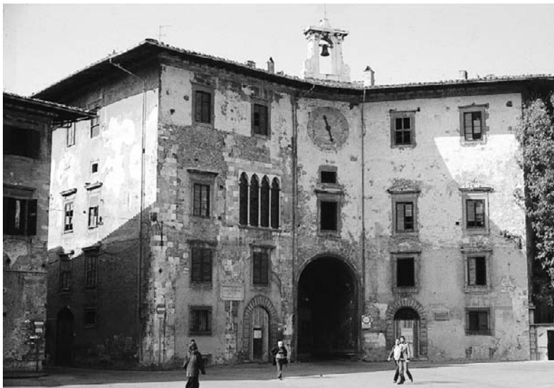
Figure 8.14 The early seventeenth-century elevation of Palazzo dell'Orologio in Pisa was taken by Brandi as an example of incorrectly conceived restoration. The remains of the reconstructed Gothic window represent a feature from a past phase now in ruin. It would have been more correct to allow the integrity of the classical façade to prevail
