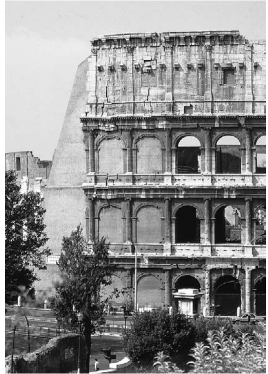
Figure 4.3 Consolidation (1806) of the eastern section of the Colosseum by R. Stern who took great care to preserve the antique fabric in the state as found
