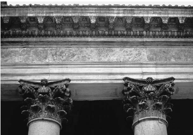
Figure 2.8 The Roman Pantheon was 'rehabilitated' as a mausoleum for the family of Pope Alexander VII Chigi, starting from 1662. The east side of the portico was rebuilt with columns and marble from nearby excavations; the papal symbol and the emblem of the Chigi family were carved on the new work
