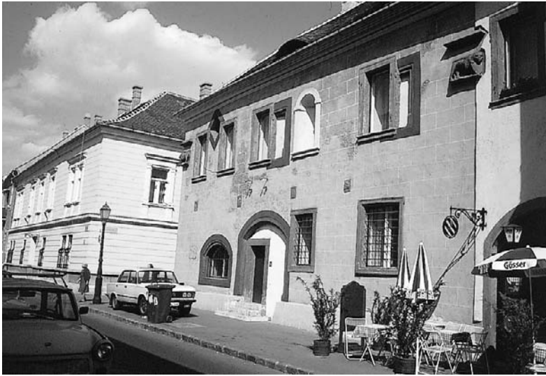
Figure 9.20 Old Buda in Budapest was rebuilt after damage in the Second World War. The policy was to display original fragments in the reconstructed buildings as a testimony of the past
