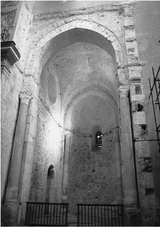
Figure 8.15 The cathedral of Cefalu in Sicily was restored by removing neo-classical plasterwork from a chapel in order to display the fragments of an earlier Norman construction – thus destroying the integrity achieved through time
