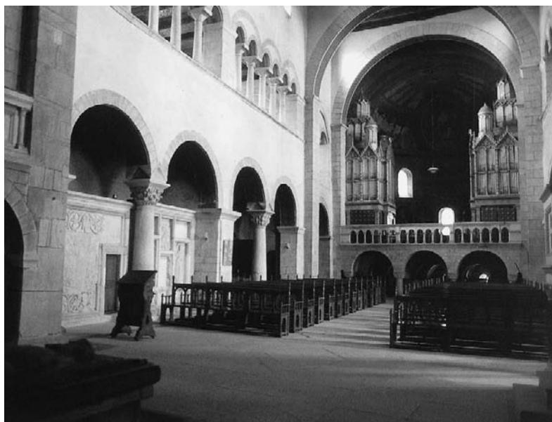
Figure 5.13 Interior of the Stiftskirche of Gernrode restored by F. von Quast, who rediscovered earlier clerestory windows under eighteenth-century wall plaster
