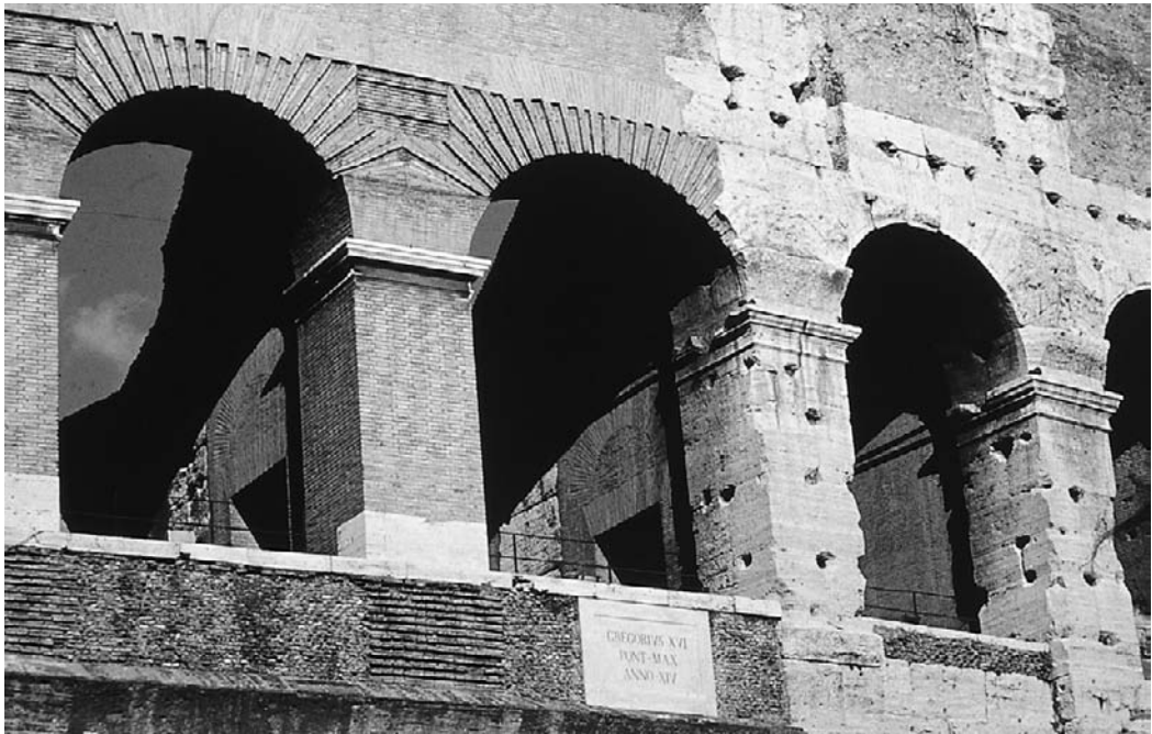
Figure 4.10 In the restoration of the southern section of the Colosseum, around the middle of the nineteenth century, L. Canina built new parts in brick in order to distinguish them from the original stone structure
