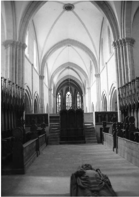
Figure 9.11 Naumburg Cathedral was seriously damaged in the Second World War, and the vaults were rebuilt under the direction of the cathedral architect, E. Schubert. The colour scheme was chosen in tonalities of grey ('Schubert grey')
