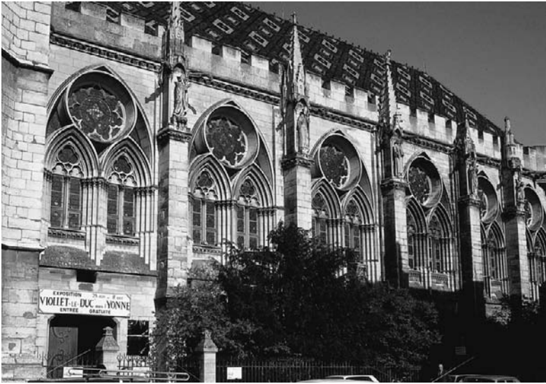
Figure 6.5 The Synodal Hall of Sens was considered by Viollet-le-Duc a perfect example that linked religious and civic architecture. The exterior was found in a ruined state, and was rebuilt on the basis of fragmentary evidence. Works were completed from 1855 through 1866
