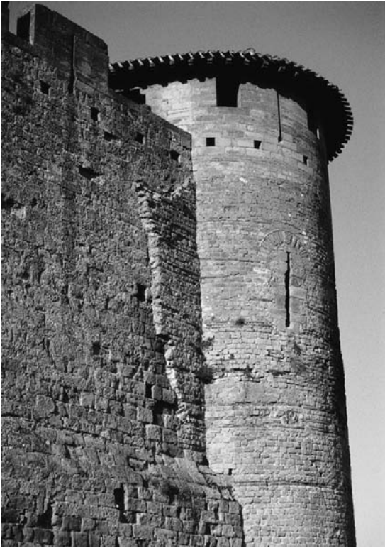
Figure 6.14 An antique Roman defence tower of the Cité of Carcassonne, reused as part of the mediaeval fortifications, and preserved in the nineteenth-century restoration. The roof has been changed in the 1960s to correspond to the supposed lower pitch of the original Roman roof
