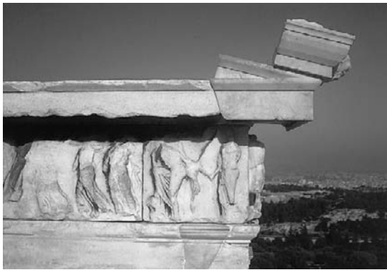
Figure 7.7 A detail of the Temple of Nike, Athens, showing the relief cast in white cement from the original in the British Museum
