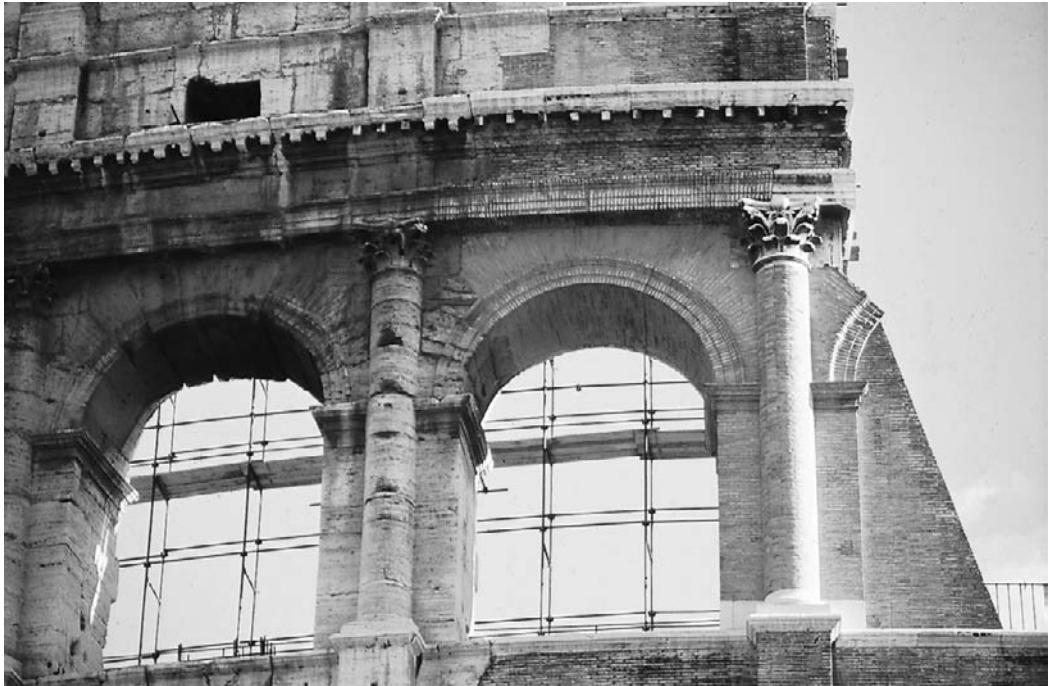
Figure 4.9 The western section of the Colosseum was restored by G. Valadier in 1824–6, who aimed at a partial reconstitution of the architectural forms. The use of brick instead of stone was justified for economic reasons
