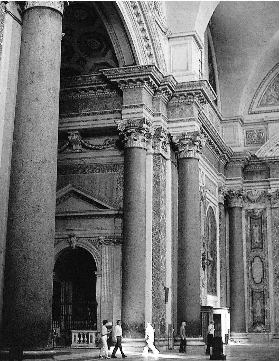
Figure 2.5 The church of Santa Maria degli Angeli was designed by Michelangelo within the ancient Baths of Diocletian in Rome, in the sixteenth century, and was subsequently modified by L. Vanvitelli in the eighteenth century
