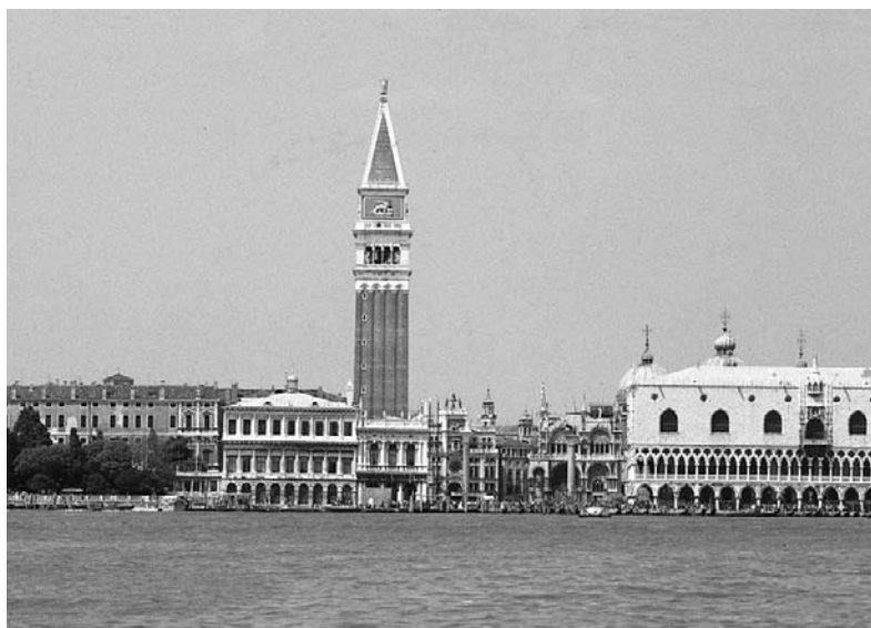
Figure 7.15 The Campanile of San Marco in Venice collapsed in 1902, and was reconstructed to the design of L. Beltrami similar to the original, ' com'era e dov'era '. The tower was considered important for the townscape of Venice
