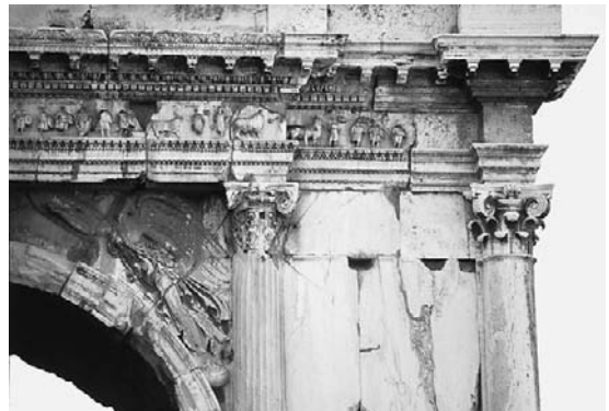
Figure 4.8 Detail of the Arch of Titus, showing new parts built in travertine without carved details, thus distinguishing them from the original in marble
