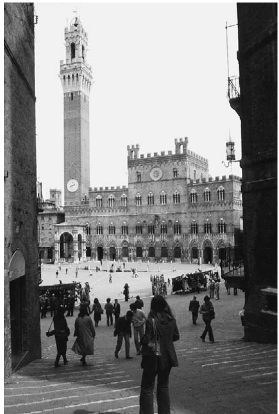
Figure 1.11 The buildings around the Campo of Siena were designed according to regulations of 1297. The upper floor of the Palazzo Pubblico (town hall) itself was built in a later period following the same pattern as the earlier construction
