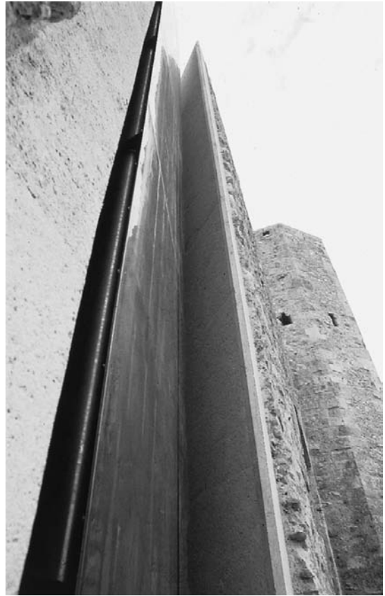
Figure 10.16 Instead of destroying the mediaeval wall that concealed the ancient Roman site in Tarragona, Spain, architect A. Bruno provided an access to restored Roman remains by making a vertical cut through the wall – as if opening the book of history. (A. Bruno, 1987–94)
