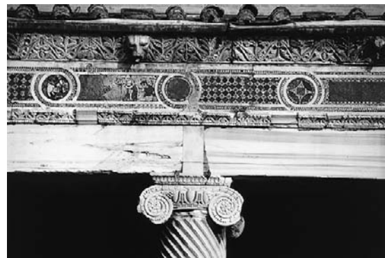
Figure 8.5 San Lorenzo fuori le mura, a detail of the reconstructed portico, a mediaeval construction using ancient spoils. New elements were kept plain in order to differentiate from the original
