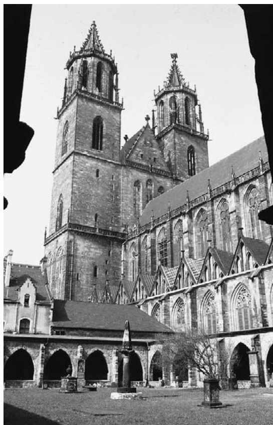
Figure 5.12 Magdeburg Cathedral in the 1980s – after yet another restoration due to damage in the Second World War
