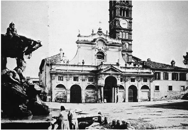
Figure 7.16 The baroque façade of Santa Maria in Cosmedin, Rome, designed by G. Sardi, was removed in the nineteenth-century restoration
