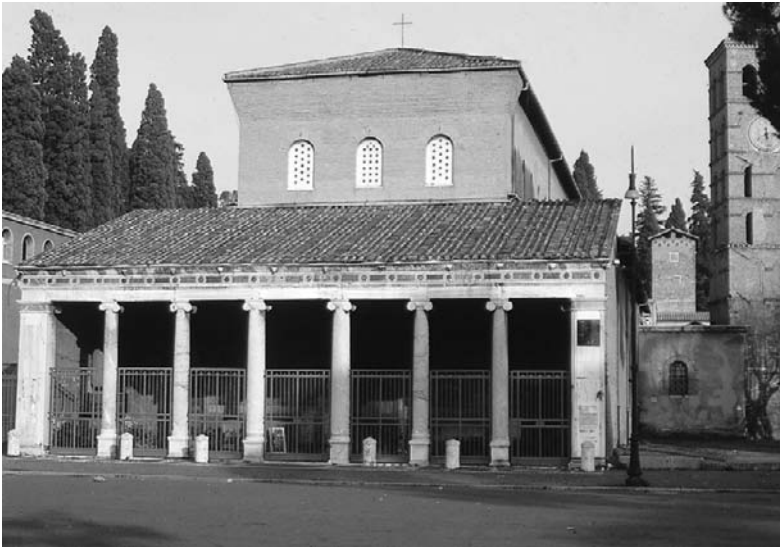
Figure 8.4 The front and the portico of the church of San Lorenzo fuori le mura, Rome, were rebuilt after destruction in the Second World War
