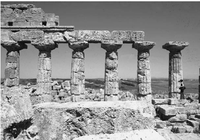
Figure 8.16 A part of the columns of Temple C in Selinunte were re-erected as ‘anastylosis’ in the 1950s. Brandi did not accept this, considering that the potential unity had already been lost also due to the deformation of elements after lying in the ground for centuries
