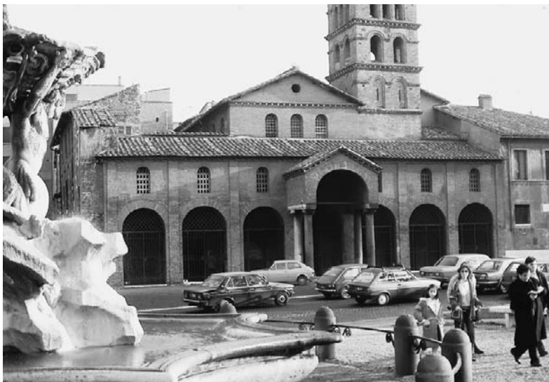
Figure 7.17 Santa Maria in Cosmedin, Rome, after restoration by G. Giovenale in 1893–9. The elevation was partly rebuilt on the basis of a hypothesis. New parts were differentiated according to principles announced by C. Boito in 1883
