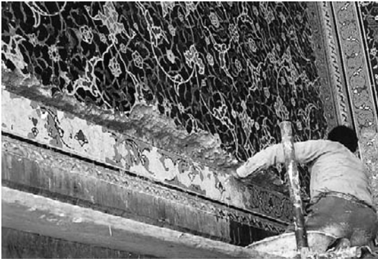
Figure 9.30 Traditional replacement of tiles at the entrance to the Masjid-i Shah, today Masjid-i Imam of Isfahan
