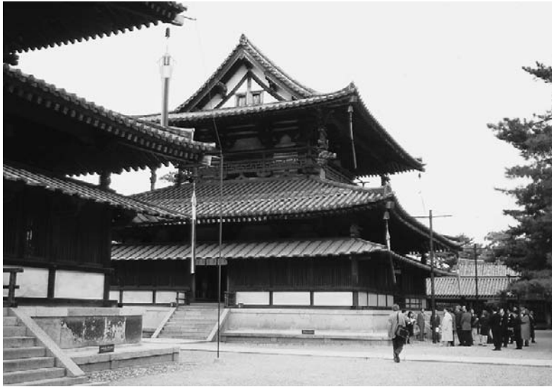
Figure 9.38 The Buddhist temple in Nara, Horyu-ji, where eventual restoration is based on the principle of replacement of decayed or rotten elements
