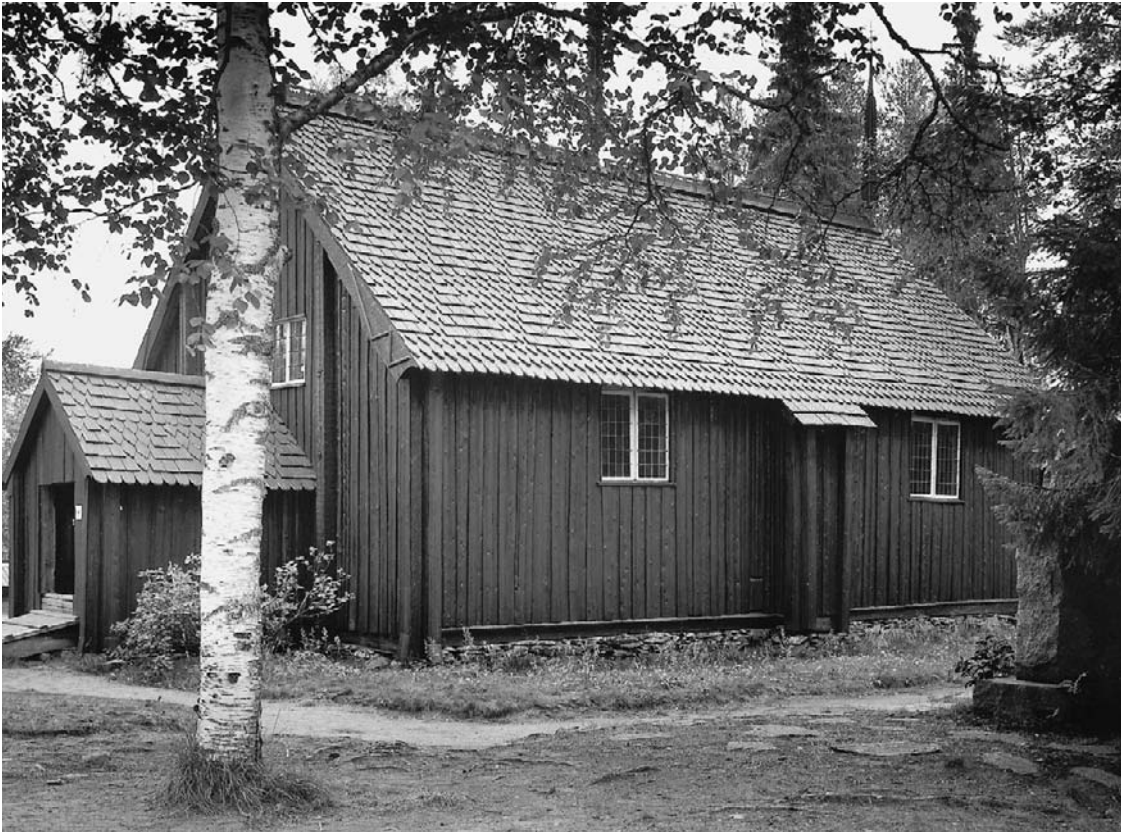
Figure 10.6 The eighteenth-century church in Sodankylä, Finland, after restoration in the 1990s with new weather boarding and roof in wooden shingles in the traditional manner. (National Board of Antiquities, Lauri Yli-Tepsa)
