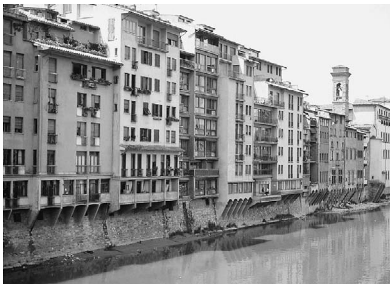
Figure 8.6 The area close to Ponte Vecchio in Florence was rebuilt in modern forms after war destruction, but keeping the same rhythm and volume as before
