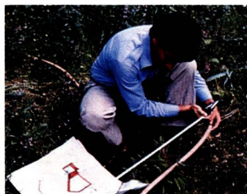
One way to lay out the general plan for your deck configuration would be to lay down nylon cord or, as illustrated, mark your proposed site with garden hose.
