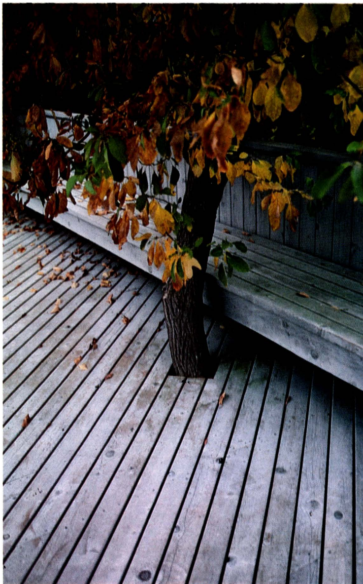
Cutouts in the decking allow trees to grow through and cover part of the deck. Care must be taken to allow a big enough hole for growth and wind sway. Never attach a deck directly to a tree, unless it's a tree house deck and is unattached to anything else.
