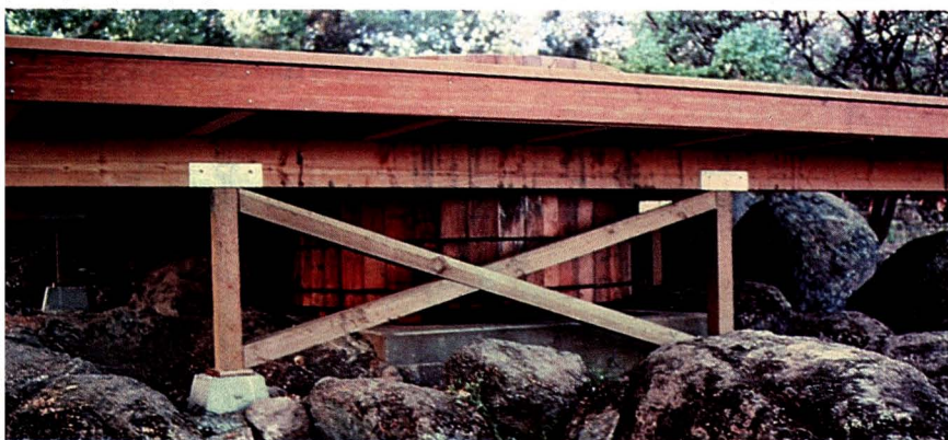
Cross-bracing strengthens a deck against lateral (sideways) movement.
