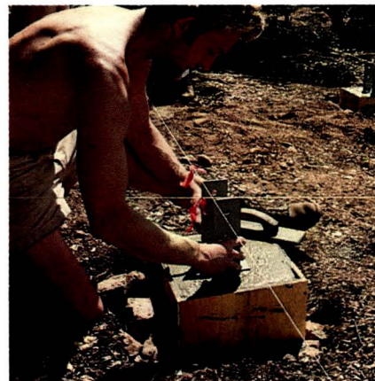
Position footing along batter boards.
