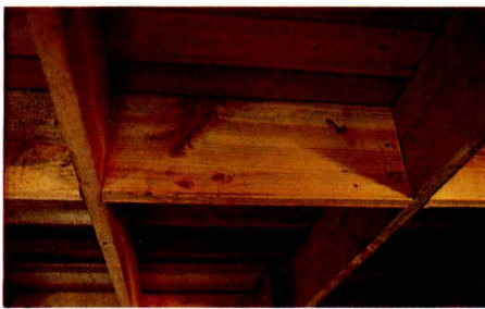
Blocking is necessary to stiffen many deck structures. Design for rock solidness as you work back and forth on the lumber sizing tables. Don't cut down lumber sizes if you want to have a solid deck.
