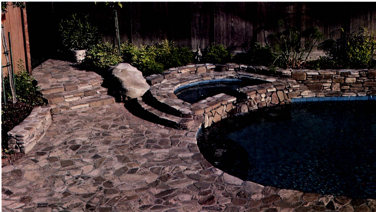
Stone paving and flagstone paving can add textural complexity and durability. Watch out, though, for rough surfaces where bare feet or bodies are apt to be, as at pool side. Large rocks, in such instances, can blend well with smaller ones to soften edges.
