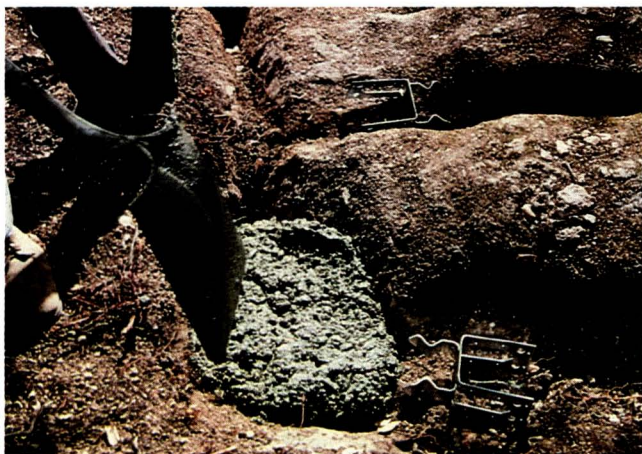
Prepare the site and pour concrete. Have fittings handy.
