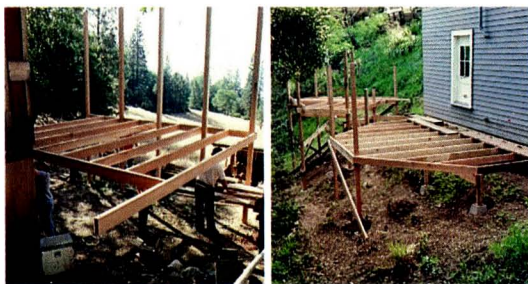
Deck structures under construction.
