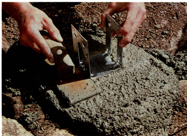
Position and level footing.
