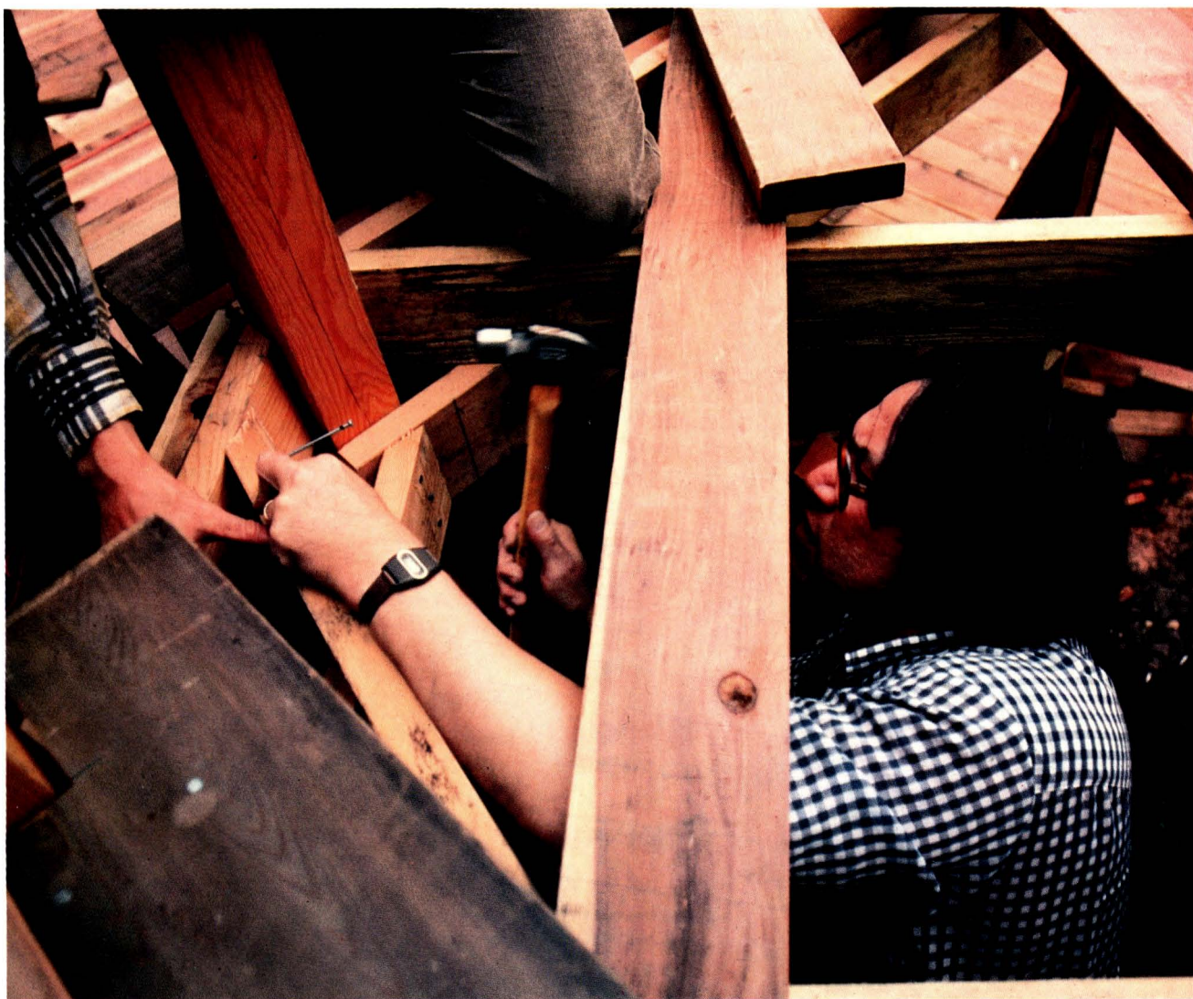
A builder sometimes finds it necessary to work in awkward spaces, especially when joining joists to beams.
