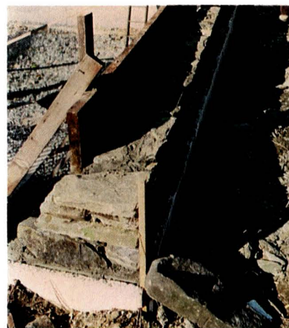
Formwork for a concrete wall must be sturdy and can be three-dimensional.
