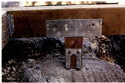
Saddle fittings or pre-cast piers provide alternate supports for decks.
