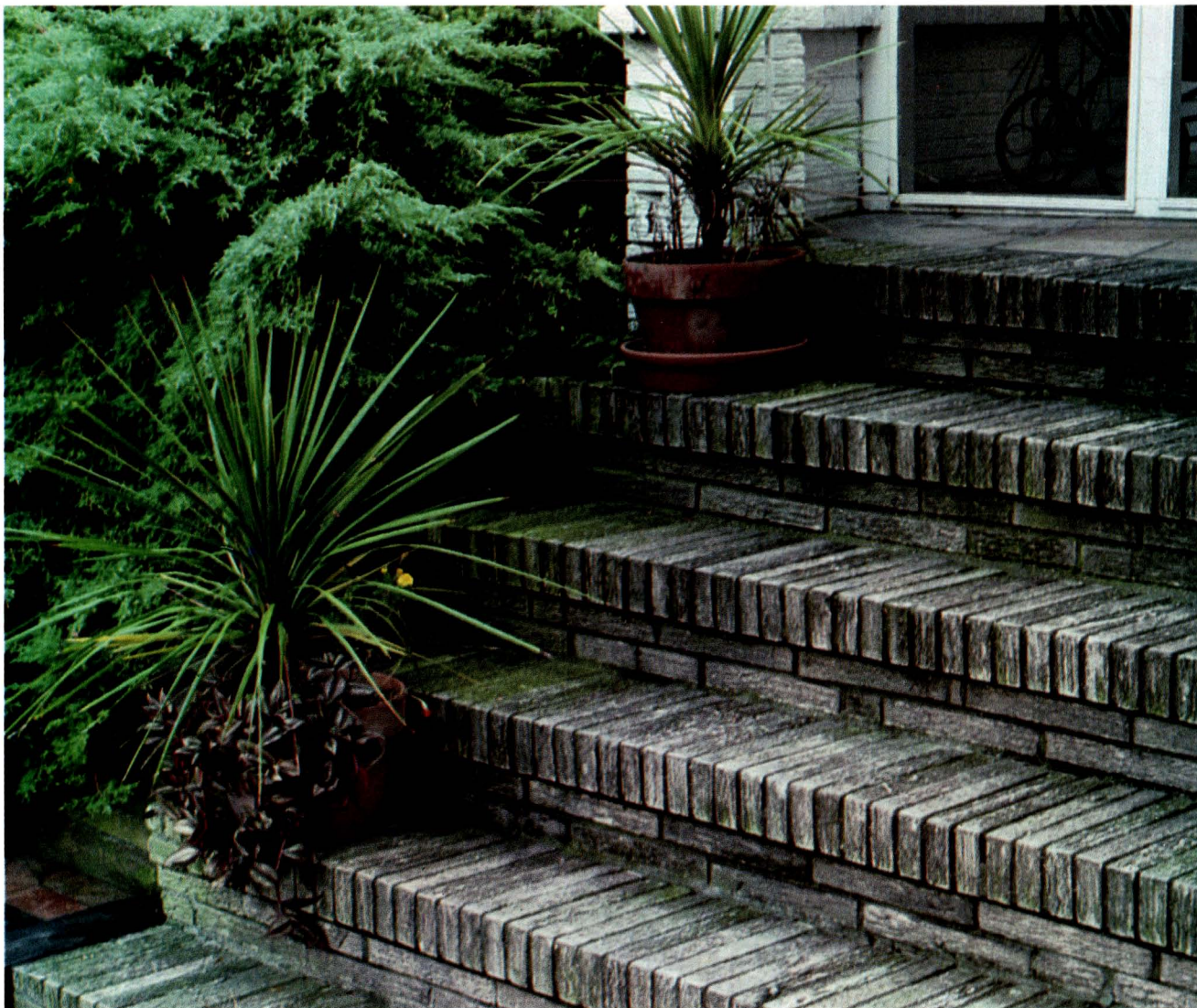
Patio and deck steps should have uniform treads and risers, and be grouped at least two per set. Single steps are hard to see and may be dangerous whether or not they are shallow or deep.
