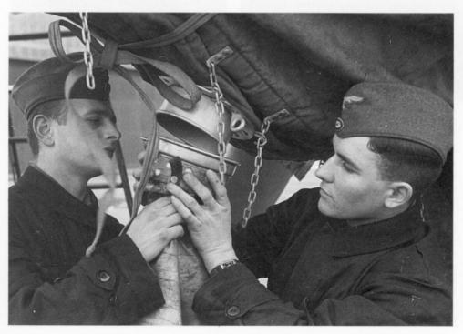
Left: The Fliegermütze of the type worn by Men and NCOs. Two ground mechanics attach the nozzle of a hot-air generator to the underside of an aircraft engine. Pumping hot air around the engine assisted starting during cold weather.
