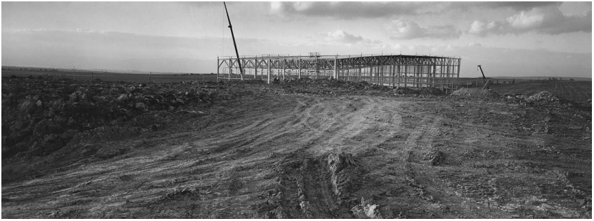
Plate 7.2 Nemak aluminium factory, construction site © Ibra Ibrahimovič
