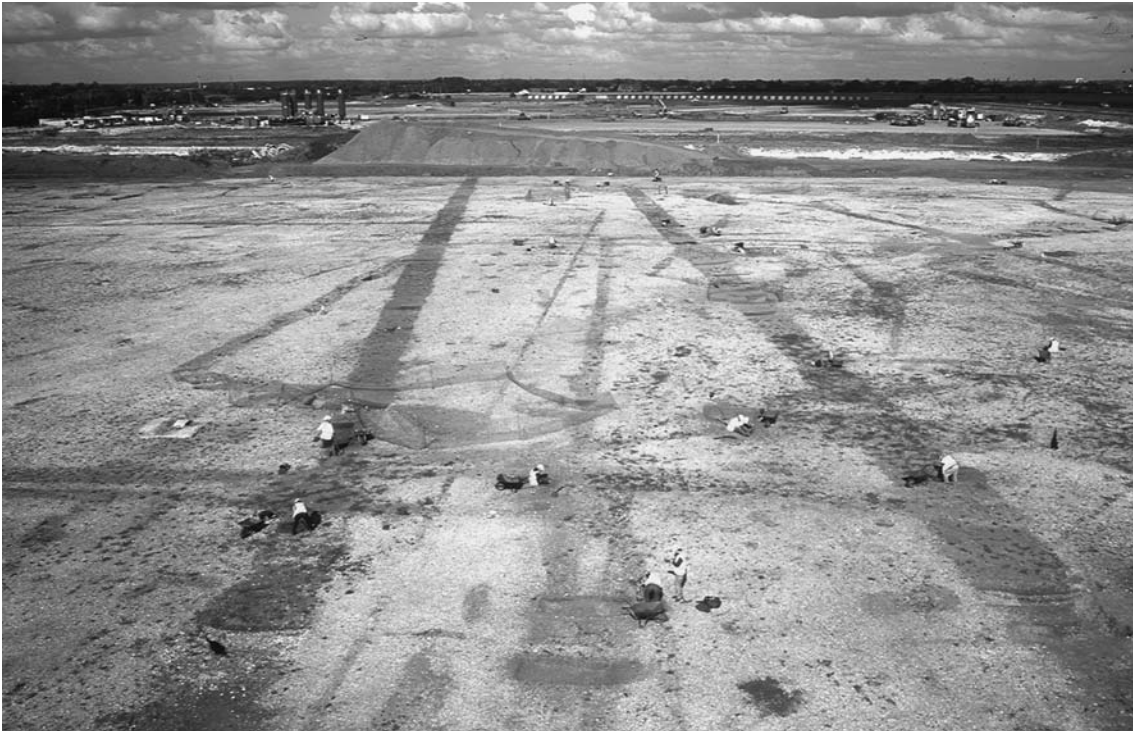
Figure 2.4 Excavations on the site of Heathrow Terminal 5
