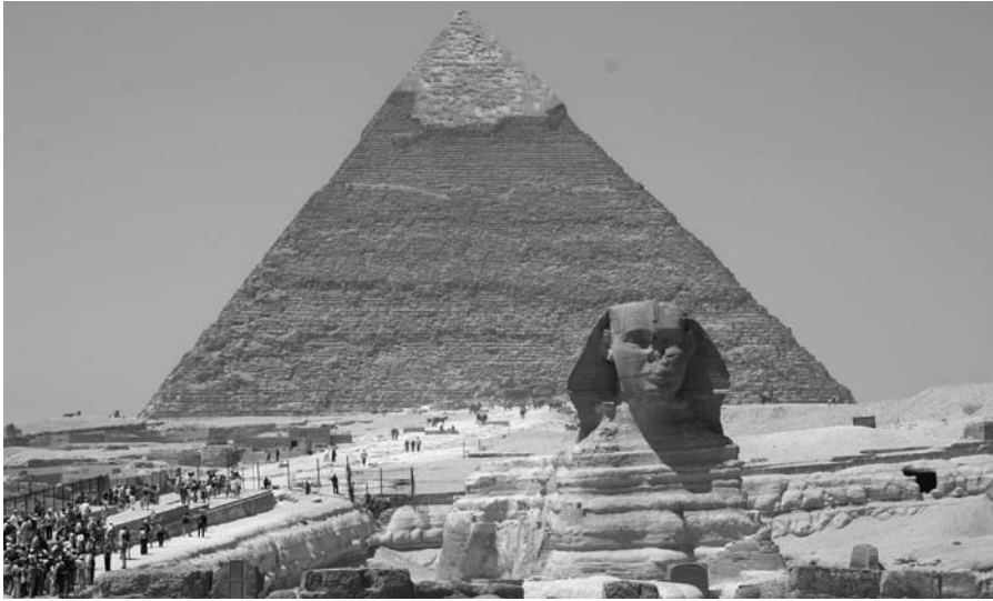
Figure 10.4 Climatic damage to the Sphinx
