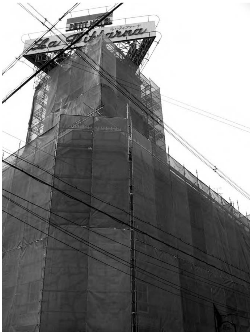
Figure 5.5 Hotel La Tiffarna under reconstruction, Uehonmachi, Osaka.
