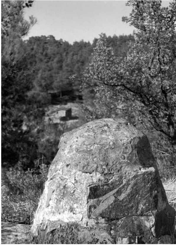
Figure 5.3 Masonry and plaster forest cairn, with part of Karterouni settlement visible behind it. Height of cairn: 1.0 m. Photograph: Michael Given.
