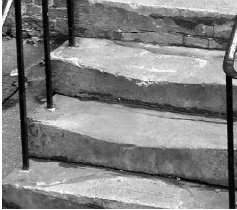
Figure 5.1 Worn stone steps indicating heavy use. (Photograph by the author)
