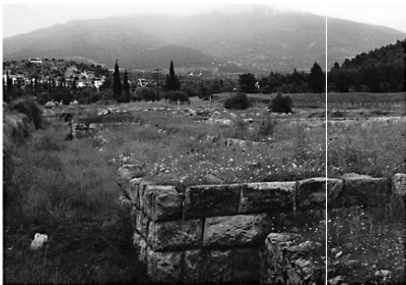
Figure 4.7 The channel of the western stream and the ashlar masonry of the western section of the enceint wall, which served also as a retaining wall.
