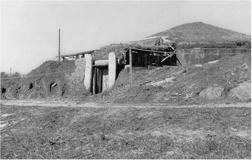
Figure 2.3 1930s New Deal relief project: reconstruction of the prehistoric earthlodge at Ocmulgee National Monument, Georgia, Photo courtesy of National Park Service.
