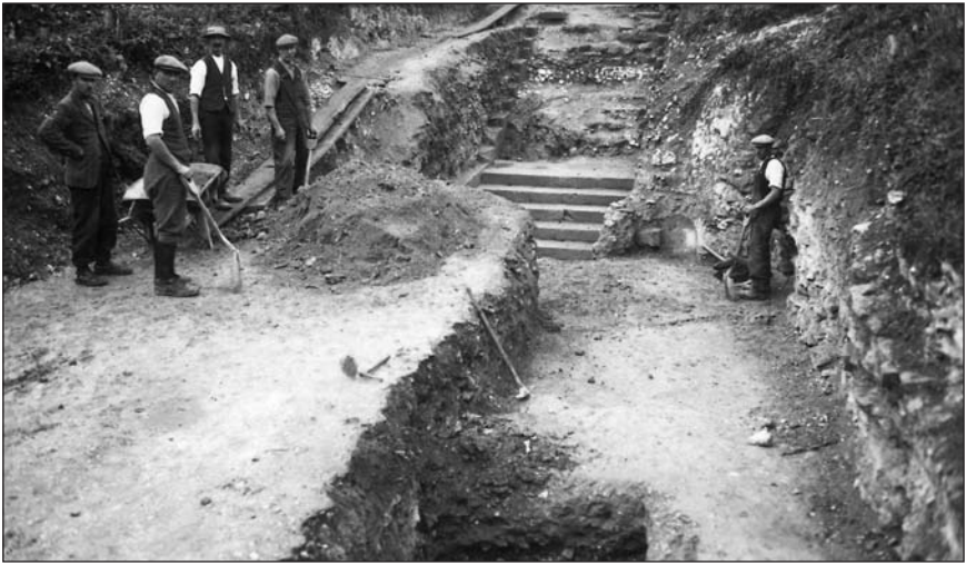
Figure 3.5 Excavations in the royal wine cellars at Clarendon Palace in September 1938, directed on site by John Charlton. The lower flight of stone stairs was found to be intact and, in the photograph, the original floor surface of the eastern flank of the northern cellar has just been exposed by workmen. The work was halted at the outbreak of war in 1939 and remained unpublished for almost fifty years. (Photo: Clarendon Archive, King Alfred's College, Winchester).
