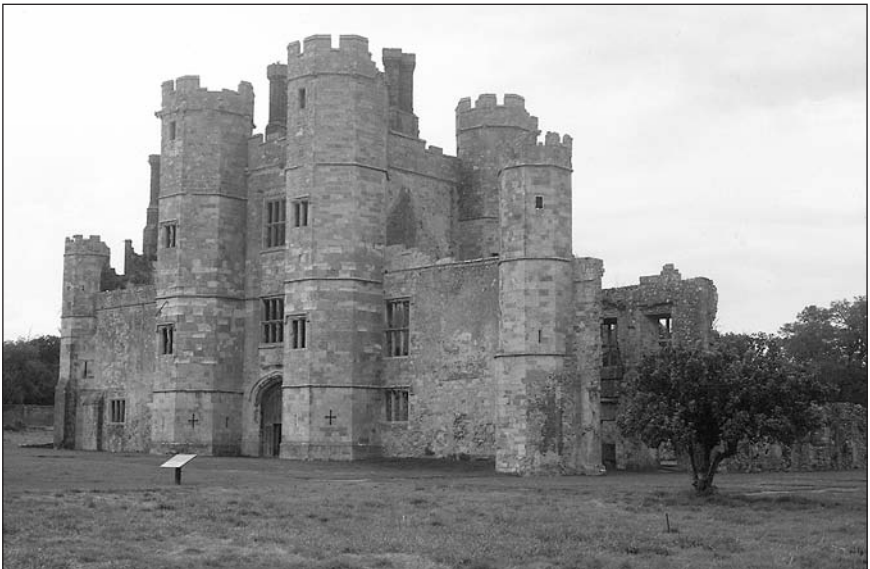
Figure 3.2 The Premonstratensian abbey at Titchfield, Hants. Converted by Thomas Wriothesley 1537–42 and largely demolished in 1781. Wriothesley inserted this turreted gateway into the monastic nave. The site was taken into guardianship in 1923. (Photo: author).
