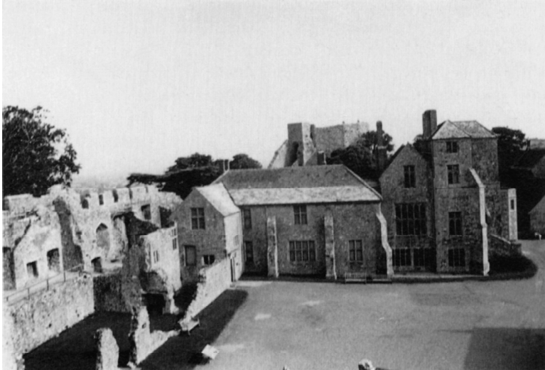
Figure 6.1 Carisbrooke Castle, Isle of Wight. The enclosure castle consisted of a large space contained by curtain walls, within and against which halls and ancillary buildings could be constructed. To the left of the picture are ruined buildings against the curtain wall; in the background is the earlier shell keep (c. 1136) perched on a motte; in the middle ground is the residential block built by Isabella de Fortibus (c. 1262–93), with later additions at both ends of the block.
