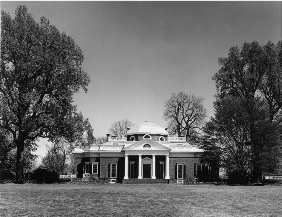
Figure 18.5 Thomas Jefferson’s Monticello, Virginia (begun 1771, remodelled 1793–1809). Photograph courtesy of Robert Lautman/Monticello/Thomas Jefferson Foundation Inc.
