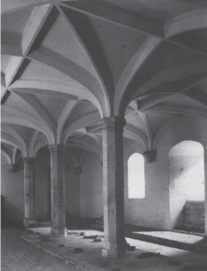
59 Hampton Court (Greater London). Cellar under the Great Watching Chamber. The raised platforms carried racking for wine or beer barrels. (Photograph: RCHM England.)
