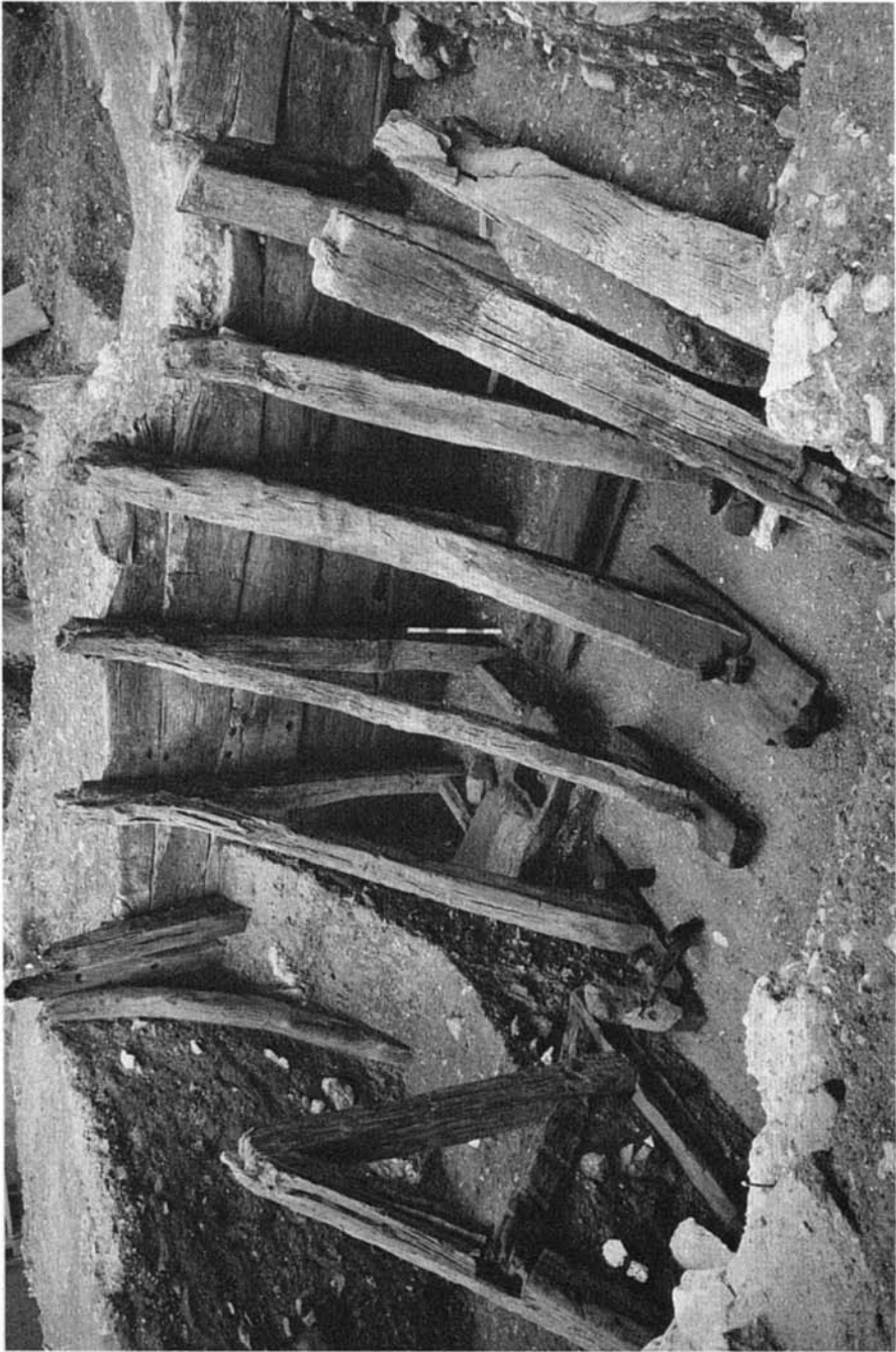
Plate 6.6 London's medieval waterfront at the Thames Exchange site: a front-braced timber revetment of the twelfth century looking north (i.e. from the contemporary river bank). The free-standing timbers in the foreground were probably part of a scissor-braced jetty which served warehouses in the waterfront area (scale 0.50m/c. 1 ft 6 ins) (Photograph: Museum of London)
