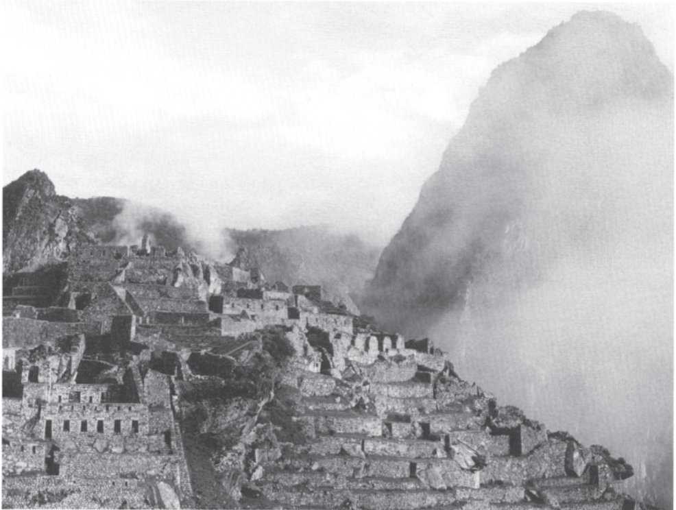
Figure 5.5 Machu Picchu, a city of the Incas in the Andes Mountains east of Cuzco, Peru. The stone terraces held soil in which crops such as maize were grown, thereby slowing erosion. Photograph taken in 1974.
