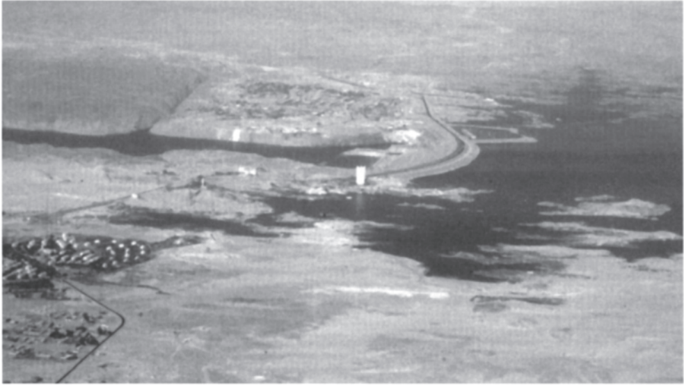
Figure 7.5 Aerial view of the Aswan High Dam on the River Nile in Egypt; Lake Nasser to the right. This dam, which ended the annual flooding of the Nile, impounds two years' flow of the river. It has been hailed as one of the greatest projects of the twentieth century and denounced as a major ecological catastrophe.
