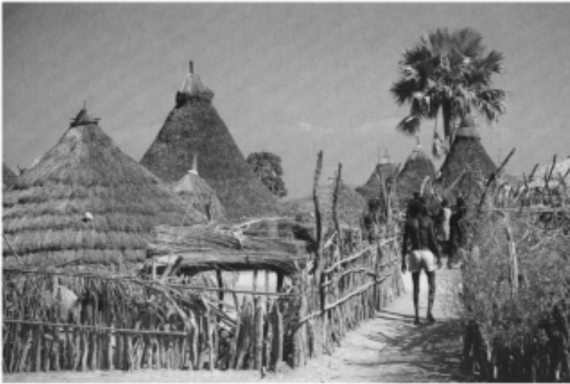
Plate 3 Three plates (3–5) show African settlements, although it is sobering to reflect that the village of Keyala, in the Equatorial Province of the Sudan, may no longer exist, for it was photographed in 1974. Comprised of materials drawn wholly from the surrounding land, this pastoral settlement comprises a series of living huts forming an agglomerated compound. The steep roofs of reed thatch repel the occasional heavy rainfall of this savanna region, while the dry-stick fences and parched ground reflect the long dry period
