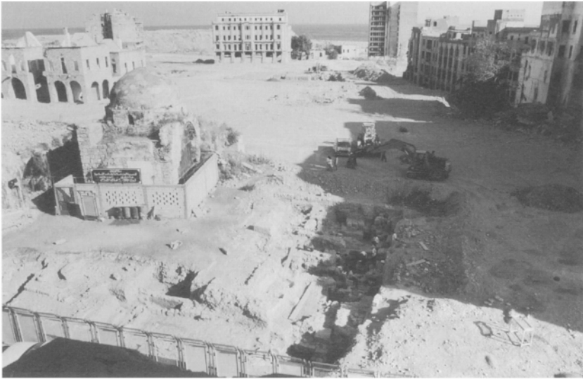
Figure 14.5 The Souks area in autumn 1994, showing retained historical buildings and the first excavations on site.
