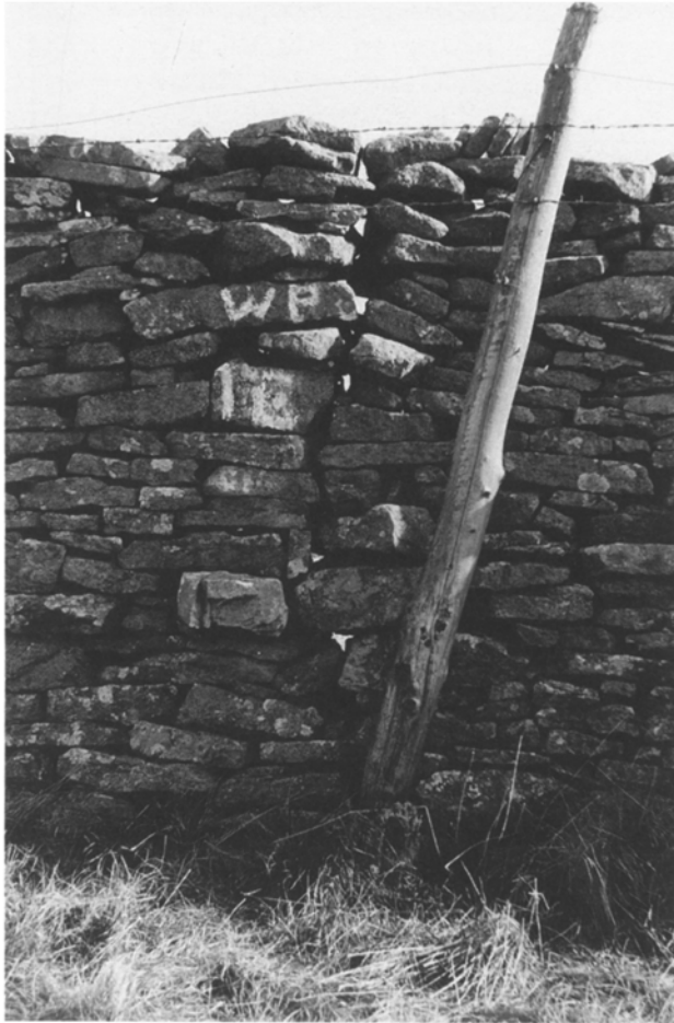
Figure 5.2 Swaledale: the stone wall separating the daleside common cow pasture and the moorland summer pasture has vertical divisions that indicate shared responsibilities for maintenance; note the recently painted initials.
