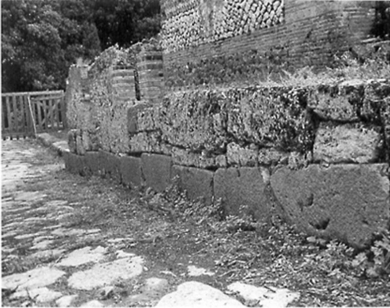
Plate 9.1 Raised pavement outside 8.2.37. Note the difference in materials used
