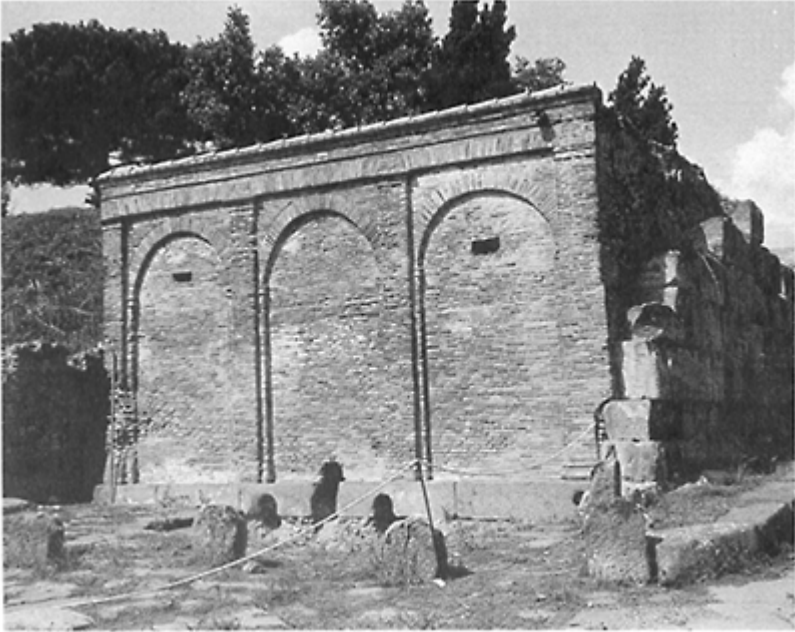
Plate 3.4 The castellum at Porta Vesuvio. Note the three pipes leaving the castellum
