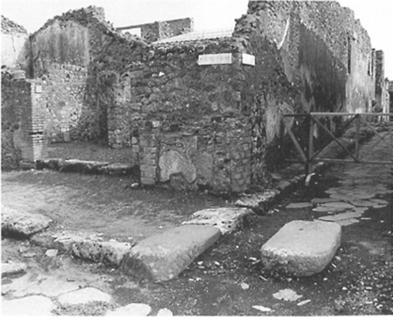
Plate 3.1 Street shrine at the north-west corner of Insula 9.8
