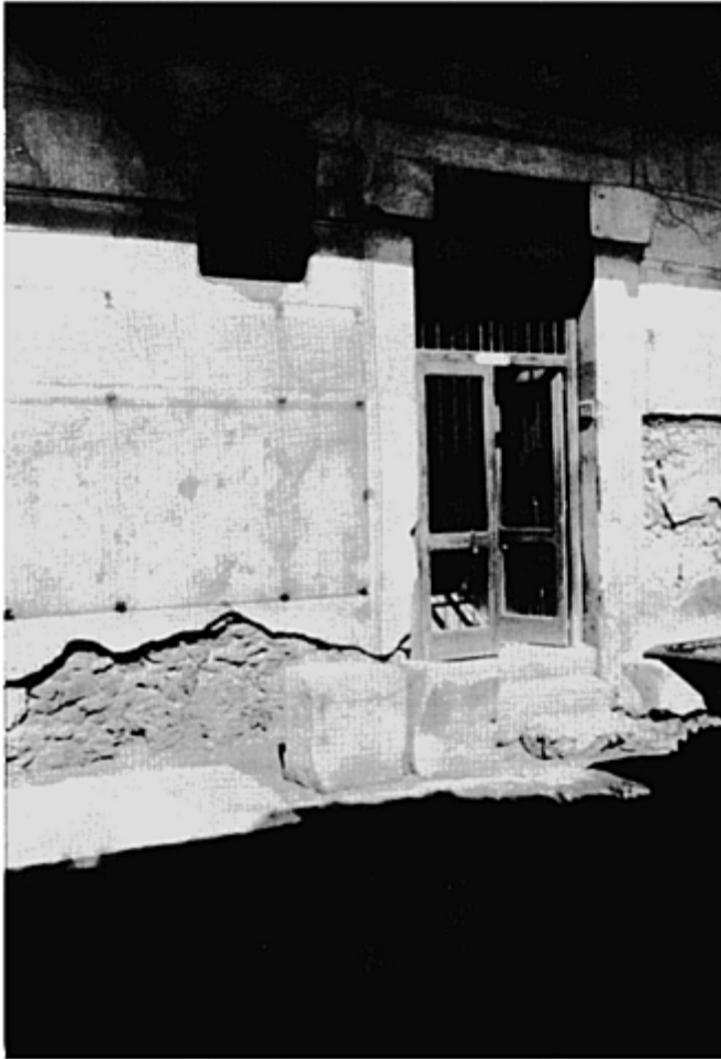
Figure 6.3 Elaboration of a doorway on the street facade
