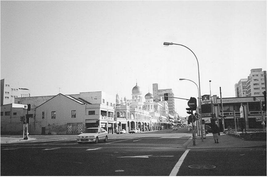
FIGURE 4.6. Grey Street mosque built at the beginning of the twentieth century in Durban.
