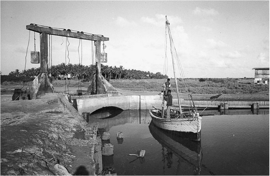
FIGURE 2.2. Sluice gate, Guyana.
