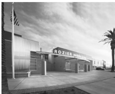
Figure 2–7. Crozier Middle School, Inglewood Unified School District, California; Dougherty + Dougherty Architects LLP (photo by Greg Hursley).
