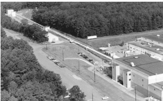
Fig. 4.5. The outside of the X-ray Calibration Facility (XRCF) at the NASA-Marshall Space Flight Center in Huntsville, Alabama. The Source Building is the small, white building at the end of the narrow pipe on the extreme left; the thin, narrow pipe is the vacuum tube. The pipe connects the Source Building with the Test Chamber that is housed inside the large building in the foreground. (Image obtained from the public image archives at NASA’s Marshall Space Flight Center.)
