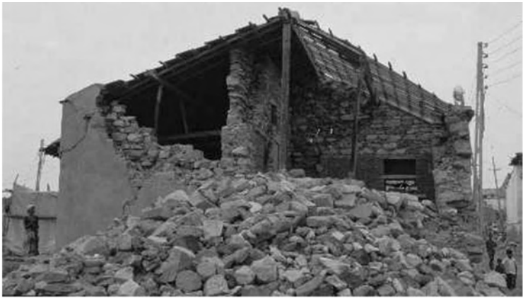
28 Buildings, not earthquakes, kill people. 400,000 poorly constructed buildings succumbed to severe ground shaking during the 2001 Gujarat earthquake in India
