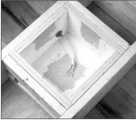
FIGURE 7.36a Recessed lighting enclosure rough-in. (Courtesy Progress Lighting)
