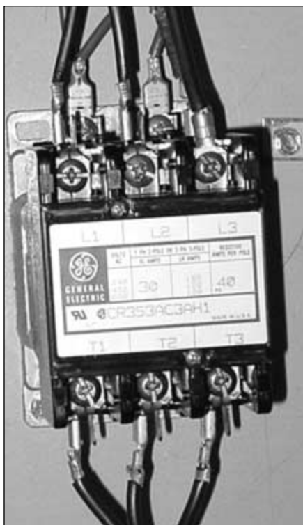
FIGURE 9.21 Three-phase contactor.
