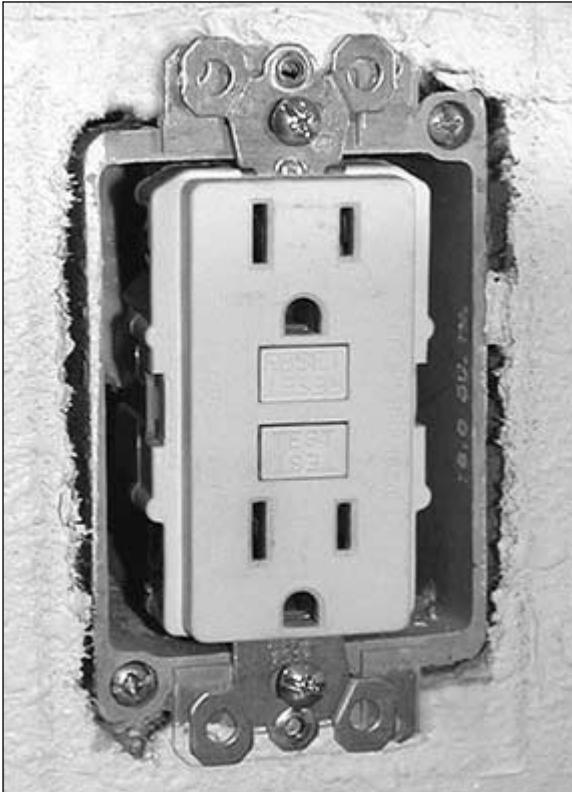
FIGURE 10.8 GFI receptacle.
