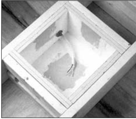
FIGURE 7.36a Recessed lighting enclosure rough-in. (Courtesy Progress Lighting)
