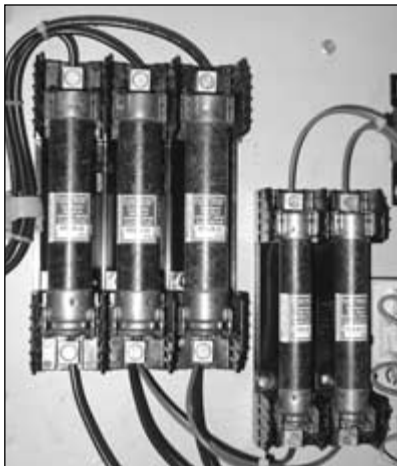
FIGURE 9.18 Fuse bank.
