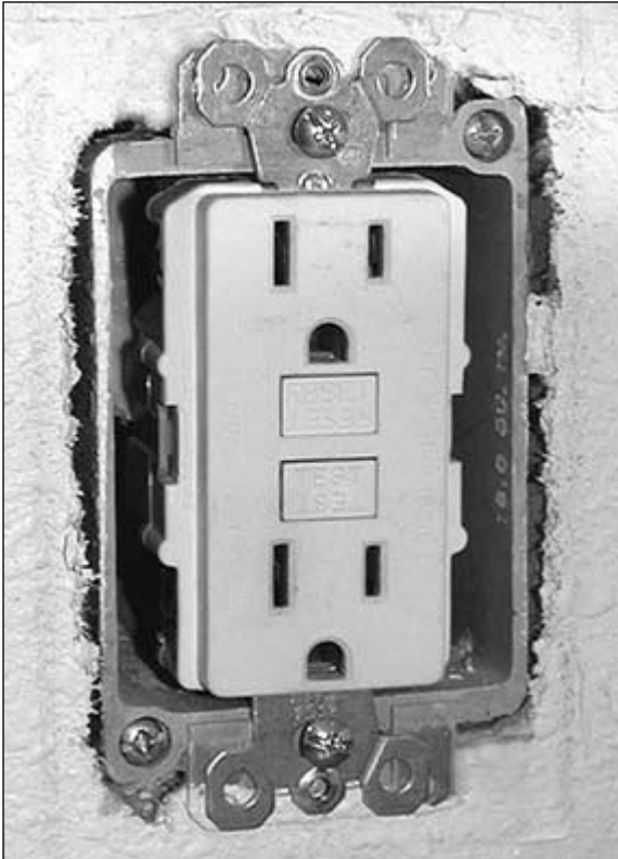
FIGURE 10.8 GFI receptacle.
