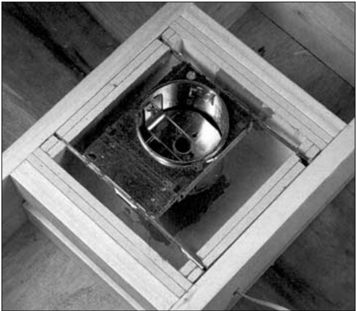
FIGURE 7.36b Recessed lighting enclosure. (Courtesy Progress Lighting)
