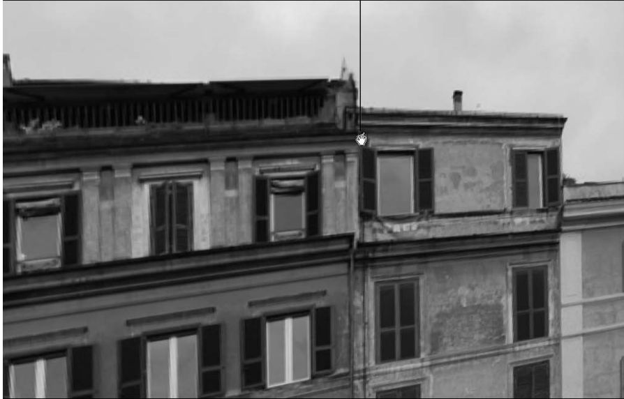
Figure 8-5: Place the pin at the corresponding corner (upper-left to upper-left, for instance) of the building in your photo.
