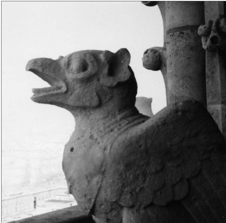
Figure 4-19: The guardrail and overlapping gargoyle are gone!
