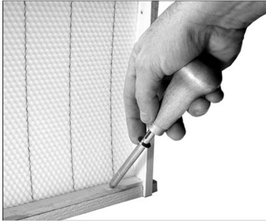
Figure 4-8: With the frame still upside- down, use a brad driver to nail the wedge strip back in place.
