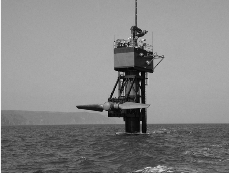
Figure 7.7 Marine current turbines “Seaflow” 300 kWe tidal current generator. Source: Marine Current Turbines.
