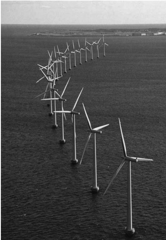
Figure 7.5 Off-shore wind farm at Middelgrunden, Denmark. Source: Middelgrunden Wind Farm. Photocopyright, Adam Schmedes, Lokefilm.
