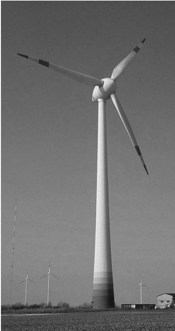
Figure 7.4 Large 4.5 MW wind turbine. Source: Enercon.
