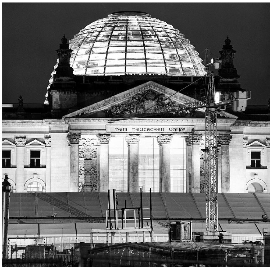
The massive glass cupola of the renovated German Parliament, opened in 1999. The British architect Norman Foster said that he intended the Parliament to be “transparent, its activities on view.” The cupola contains an observation platform “allowing the people to ascend above the heads of their political representatives.” Photograph by Hendrik Brixius.
