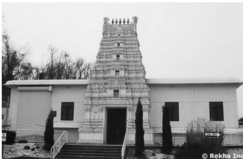
Figure 9. Building places of worship: Sri Venkateswara Temple, Penn Hills, PA 15235. A new Hindu temple in the USA, built on the South Indian pattern, which has become a vibrant social and religious centre.
