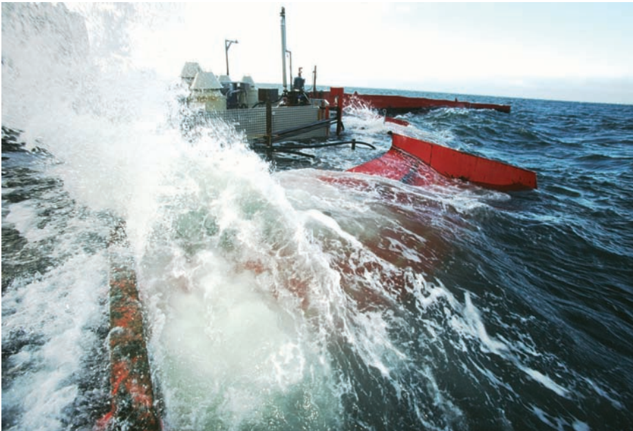
Figure 11.21 A prototype of the Wave-Dragon – a device that generates ~7 MW of electrical power from the energy available in waves is in process of installation off the coast of southwest Wales, near Milford Haven. Waves break as they rise up a ramp facing them and enter a reservoir creating a small head. Energy is generated by running water down through turbines lower in the structure. The turbines are the only moving parts.
