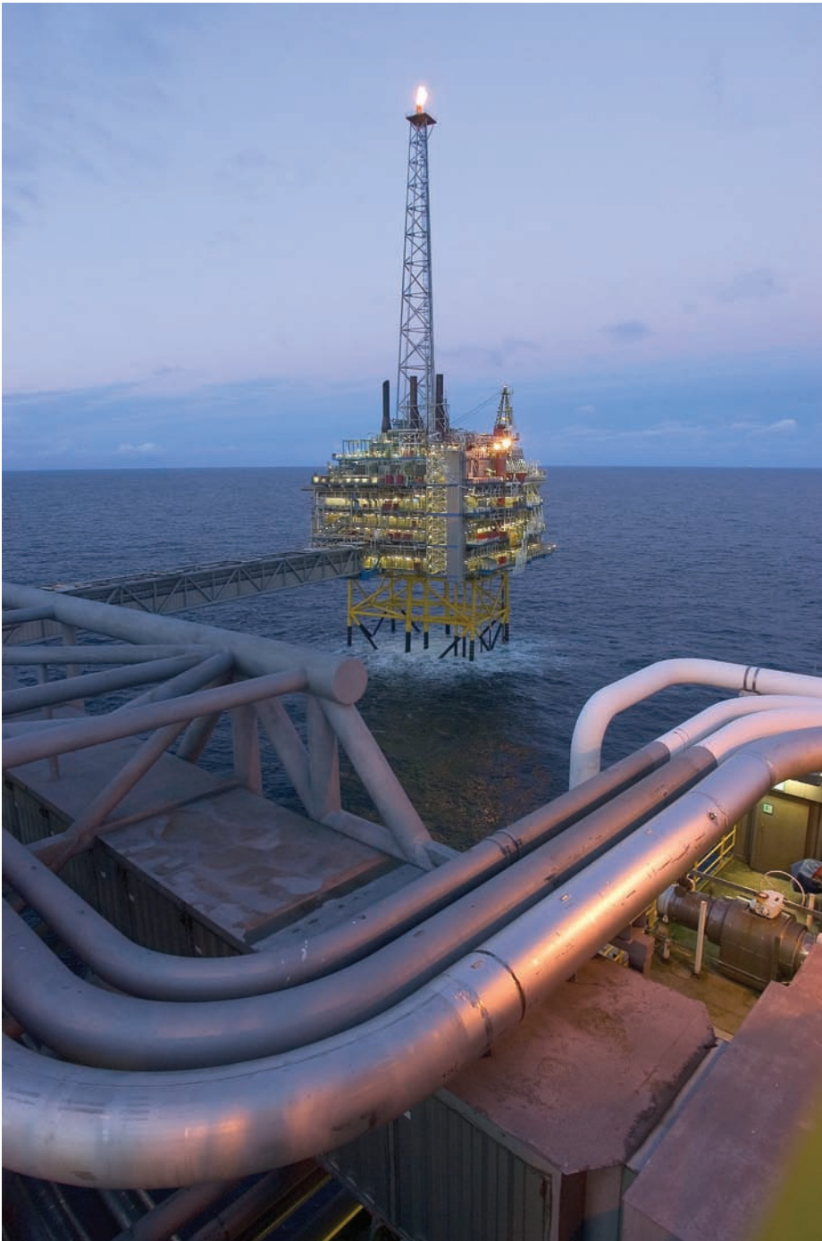
StatoilHydra's Sleipner T gas platform off the Norwegian coast which is sequestering one million tonnes of carbon dioxide per year.
