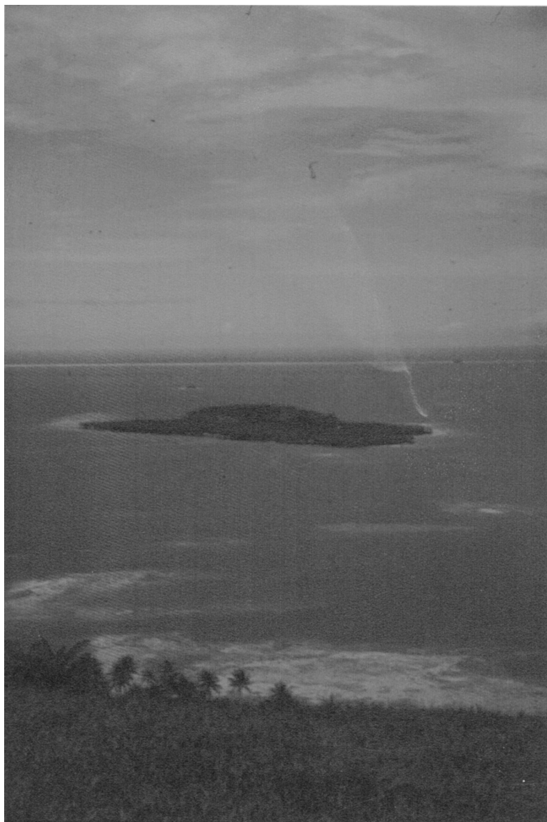
Fig. 7.5 Etten Island, Chuuk Lagoon: part of the fringing reef of Etten was covered by Japanese engineers in order to create an aircraft runway and this gives the island a form resembling a floating aircraft carrier.
