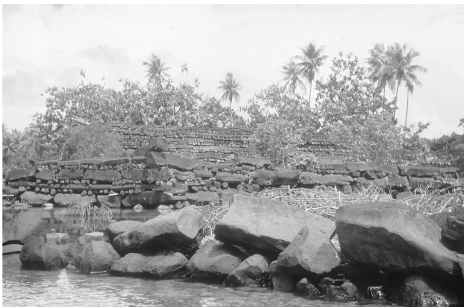
Fig. 7.11 Nan Douwas: a view from inside the breakwater entrance.
