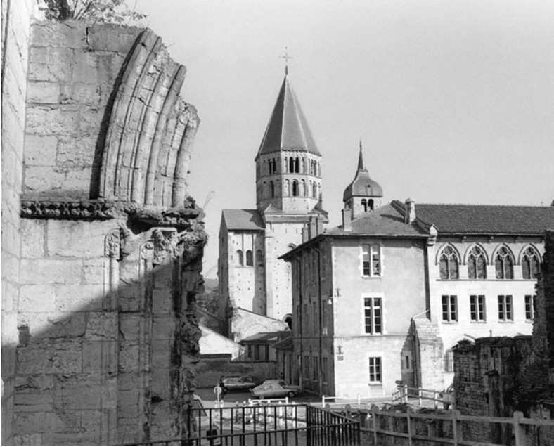
12. The abbey of Cluny, France, showing the ruined south transept.
