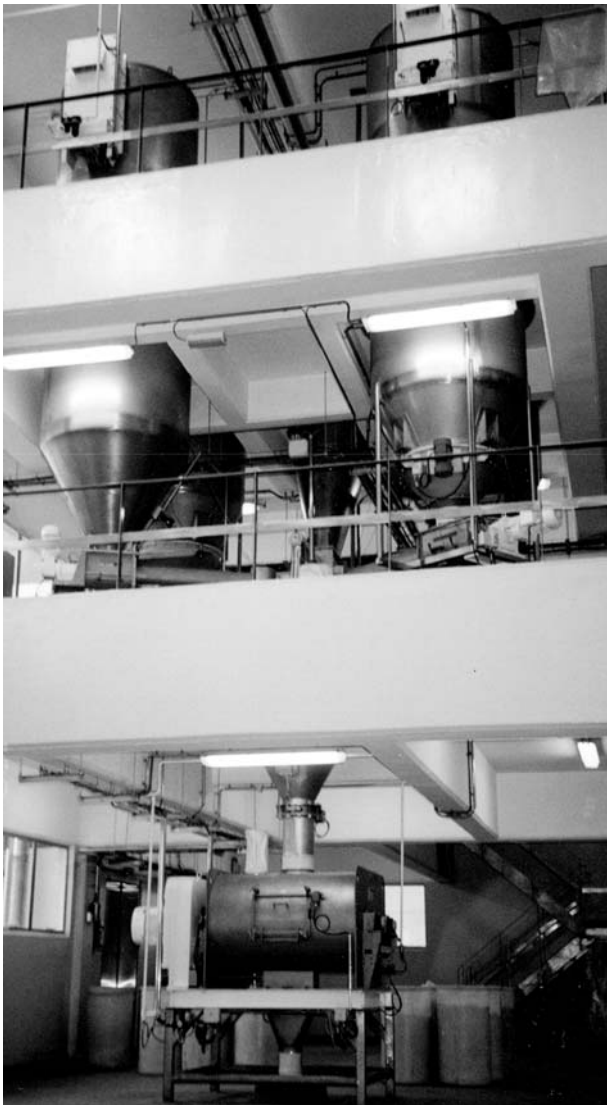
FIG. 21-52 Classical automated batch mixing installation. The components are stored in small silos shown at the top of picture. The materials are extracted from these hoppers in a downstream weighing hopper according to the recipe. Once all components are fed into this weighing hopper, a valve is opened and the exact batch falls into the downstream batch mixer.
