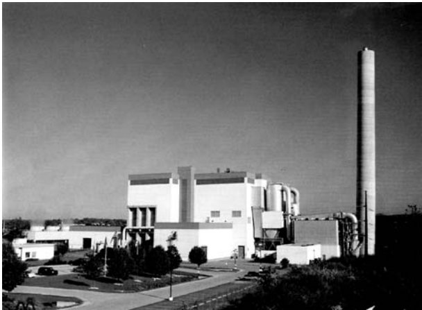
FIG. 22-52 1200-tons/day MSW plant of Montenay Montgomery.
