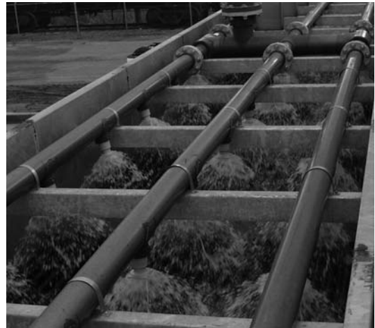
FIG. 12-8j Nozzles spraying onto wetted tube bundle in a WSAC unit.
