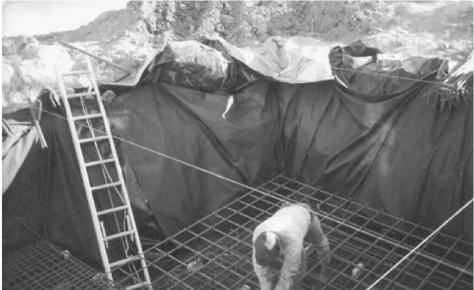
Figure 7.31 Photograph of lined foundation excavation.
