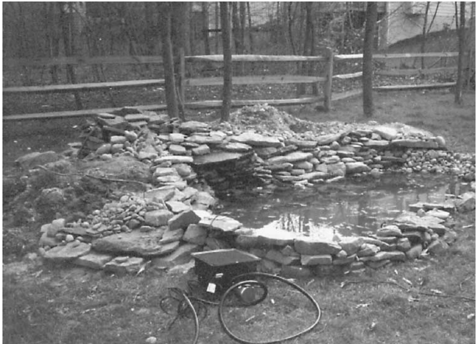
Figure 4.68 Photograph of pond installation.
