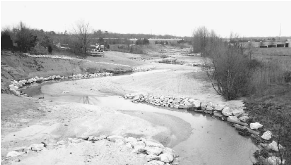
Figure 7.9 Photograph of a stream restored using the Rosgen stream assessment method as a guide.
