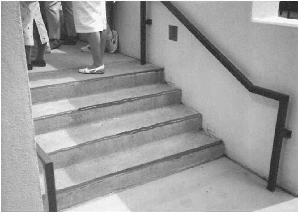
Figure 4.6 Photograph of stair treads with painted nosing.
