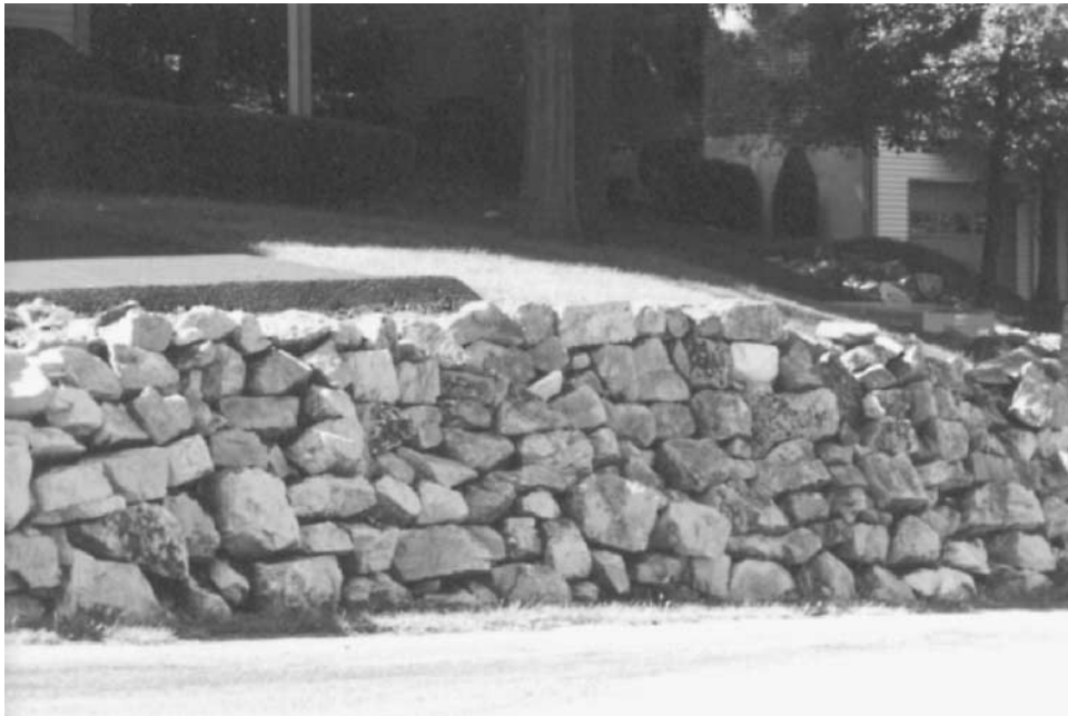
Figure 3.20 Photograph of dry laid stone wall.
