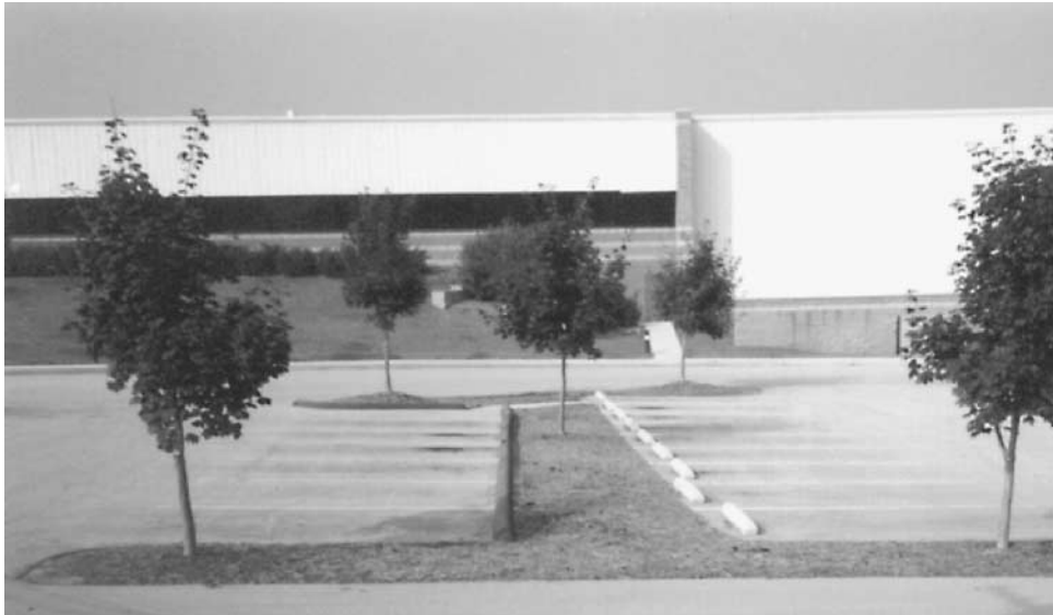
Figure 6.7 Photograph of parking lot island infiltrator.
