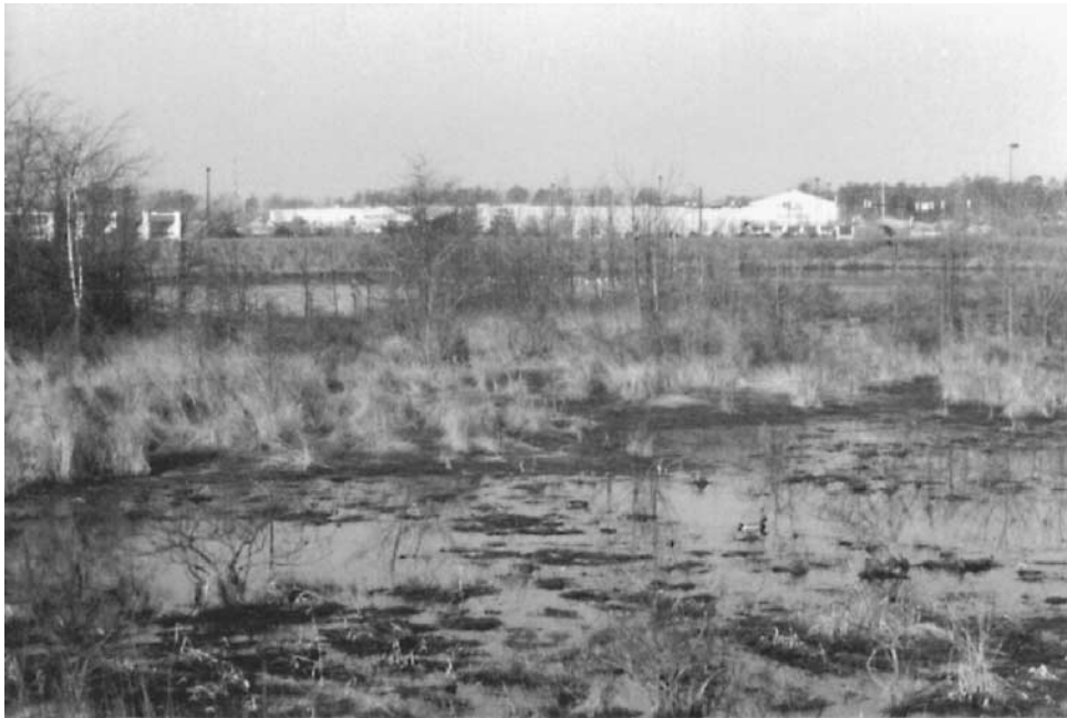
Figure 6.18 Photograph of wet pond. Note the open water beyond the shallow littoral area and the natural appearance of the pond system.
