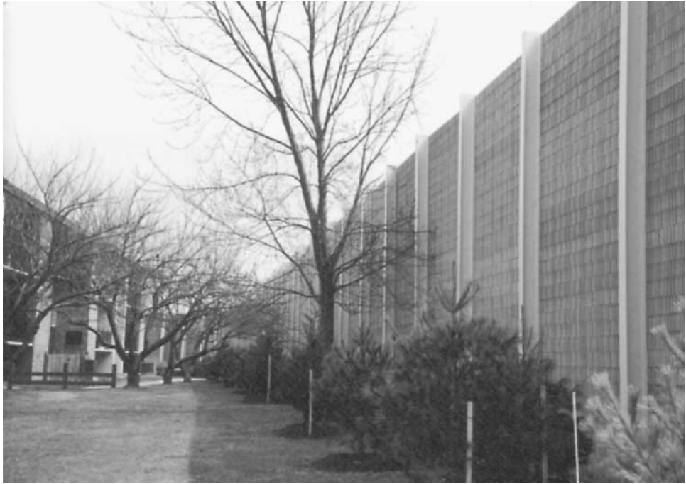
Figure 3.8 Photograph of sound walls.
