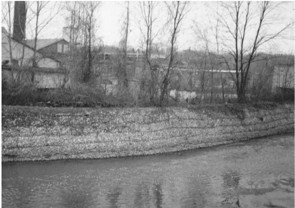
Figure 7.23 Photograph of a gabion-stabilized stream.
