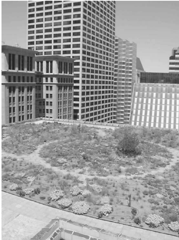
Figure 6.22 Rooftop rain garden photograph. (Used with permission of Charles Miller, P.E., of Roofscapes, Inc.)
