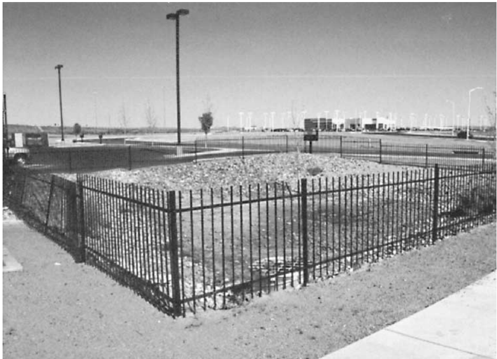
Figure 6.4 Photograph of infiltration bed in New Mexico.
