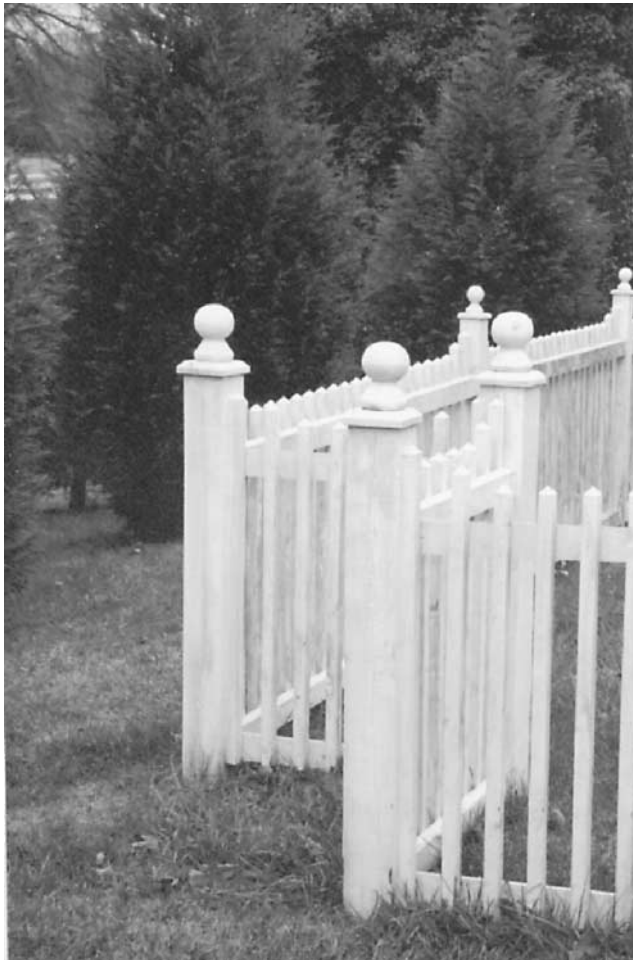
Figure 4.53 Photograph of picket fence corner detail.
