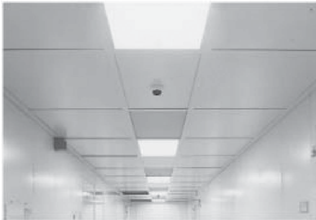
FIGURE 9 A suspended ceiling utilizing lay-in panels and lay-in lighting troffers. A variety of cleanable materials can be used for the panels. The lay-in lights should be of a design that will provide appropriate service based on the cleaning protocol to be used. (Courtesy of CleanTek.)
