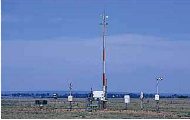
Figure 2-12. ASOS Station Installation.
