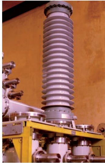
Fig. 5.16: Gas-to-air termination with composite insulator housing
