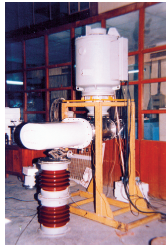
(b) Leakage Current Test
