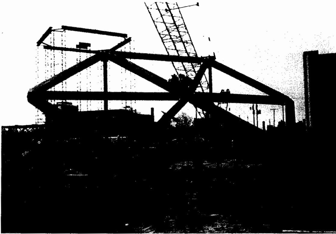
Figure 7.26 Start of ground assembly of dome—Minneapolis Convention Center.
