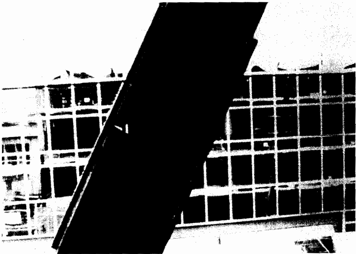
Figure 7.17 Adjustable midheight splice of bracing diagonal—Plaza Seven.
