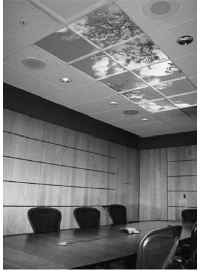
FIGURE 26 A conference room with artificial skylight made up of backlit ceiling image tiles. (See also color insert.) (Courtesy of The Sky Factory, LLC. )
