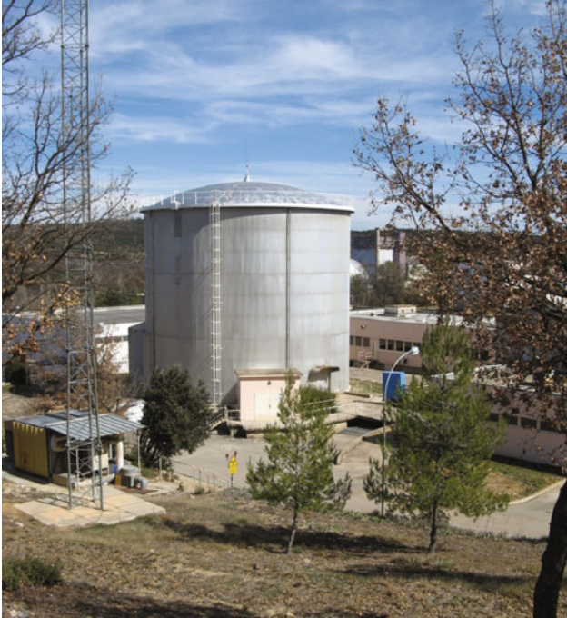
▣ Figure 40 View of MASURCA reactor containment
