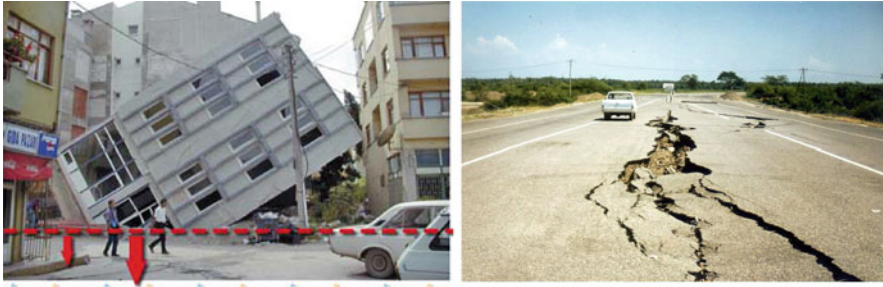
Figure 184 Physical damages of earthquakes
