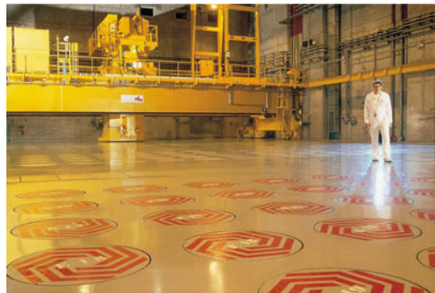
■ Figure 29 The EEV-SE facility for the interim storage of vitrified HL waste
