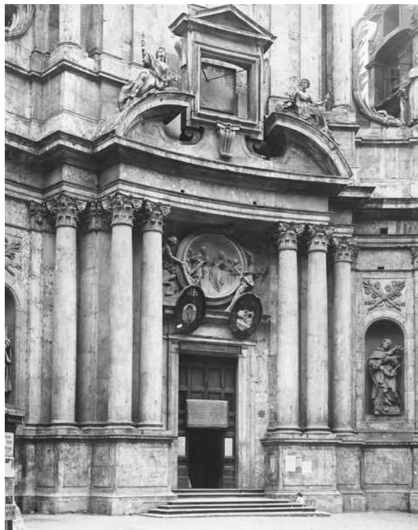
Central portion of the façade of the Church of San Marcello al Corso, Rome, designed by Carlo Fontana, built 1682–83. (Alinari-Art Reference/Art Resource, NY)
