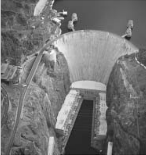
Hoover Dam (originally named Boulder Dam) is located 34 miles (54.4 km.) from Las Vegas. Hoover Dam is 726 feet high (220 meters) and 660 feet thick at its base. The dam supplies power to Las Vegas and much of the Southwest United States. © Royalty-free/Corbis. Reproduced by permission.
