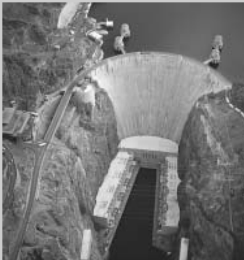
The Hoover Dam hydropower plant is driven by waters of the Colorado River. © Royalty-Free/CORBIS. Reproduced by permission.
