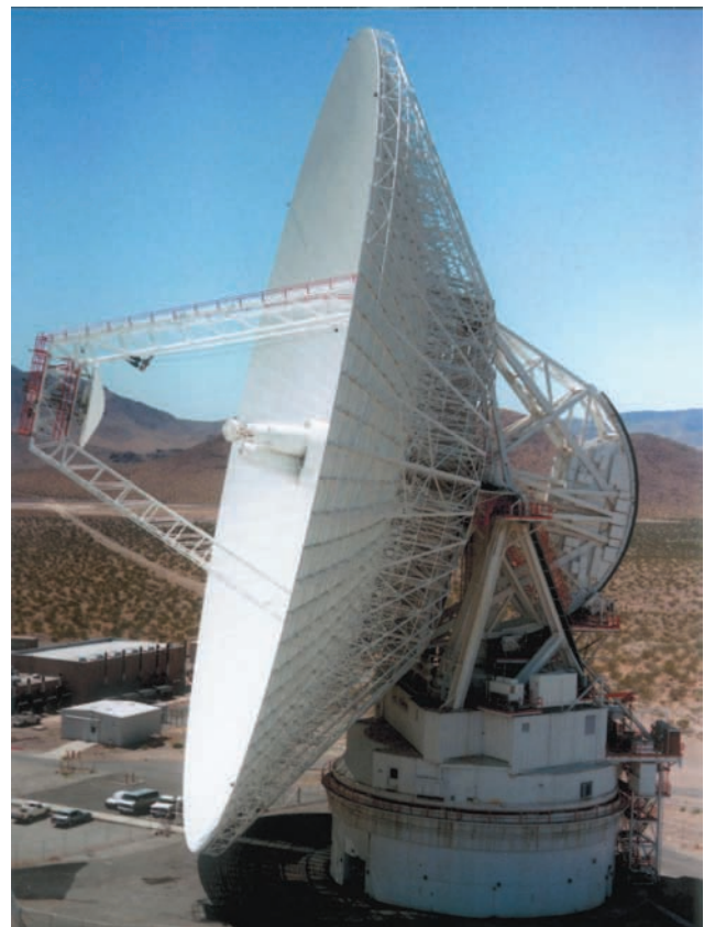
FIGURE 3 The 70-m Goldstone Solar System Radar main antenna, DSS-14, in California. The 3.5-cm planetary radar transmitter and front-end receivers are inside the lowest cone near the focus of the antenna, which is fully steerable.
