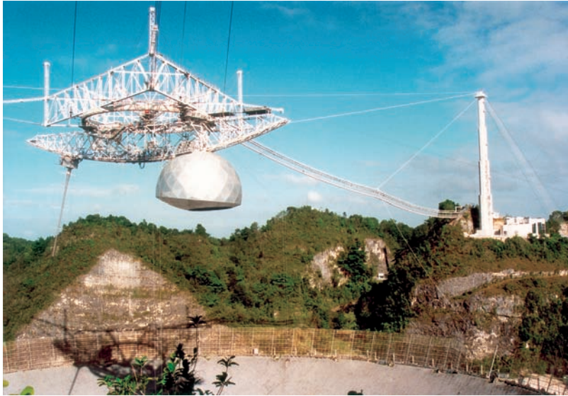
FIGURE 2 The Arecibo telescope in Puerto Rico. The triangular platform suspended above the 305-m primary reflector supports the azimuth and elevation structures that let the Gregorian feed inside the 26-m radome or the line feed point up to 20^\circ off the zenith. The S-band (2380-MHz, 13-cm) transmitter and front-end receiver are inside the radome. (Courtesy of the NAIC—Arecibo Observatory, a facility of the NSF.)
