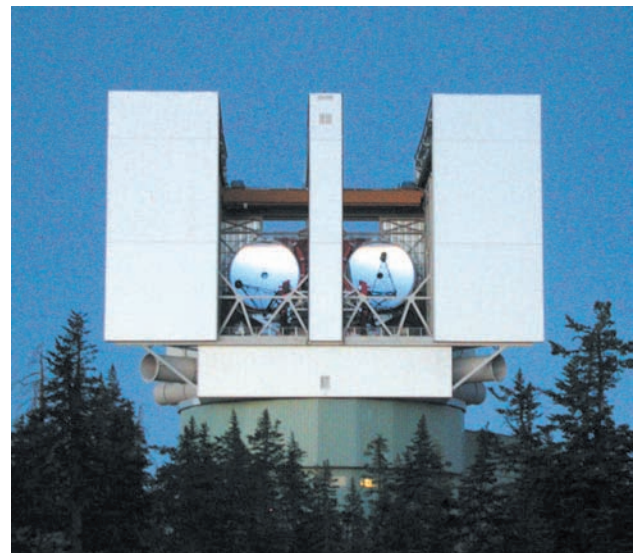
FIGURE 6d Large Binocular Telescope consisting of two 8.4-m primary mirrors. First light with a single mirror took place in 2005 and the second mirror was installed in 2006. The light-gathering power of the two primary mirrors combined is equivalent to a 11.8-m telescope. Both mirrors are on a single structure and the light from both mirrors is combined for imaging, spectroscopy, and interferometry. The combined light from the two mirrors will have the angular resolution of a 22.8 m telescope when the LBT is used as an interferometer. (Courtesy of the Large Binocular Telescope Observatory)
