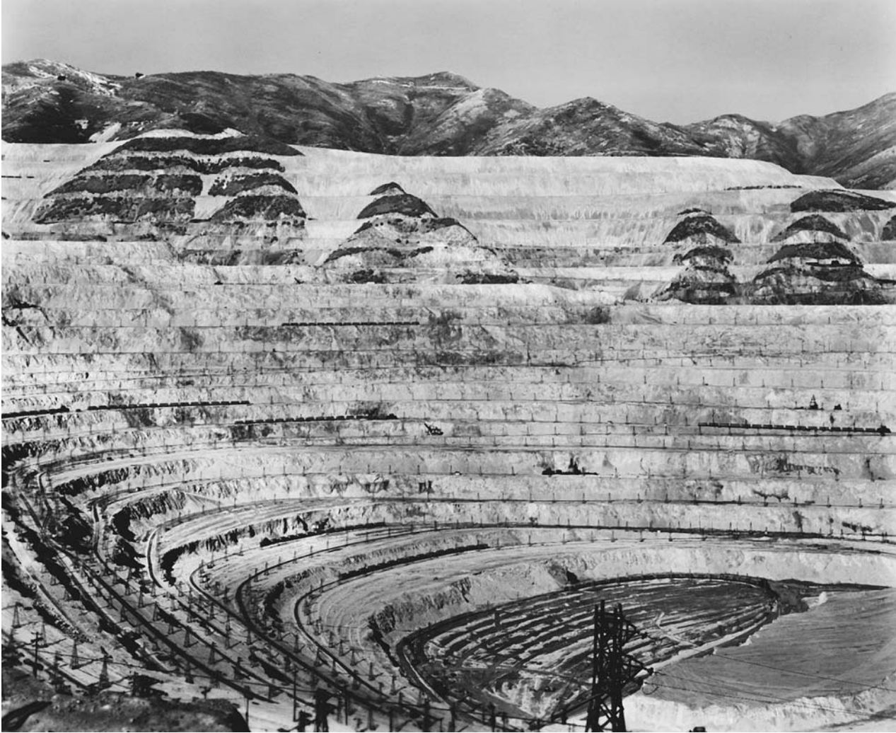
The Bingham Canyon copper mine in Tooele, Utah. This mine is the world's largest man-made excavation. Kennecott Utah Copper Corp. produces copper, molybdenum, gold, silver, platinum, and palladium from the century-old mine. (© Bettmann/Corbis.)
