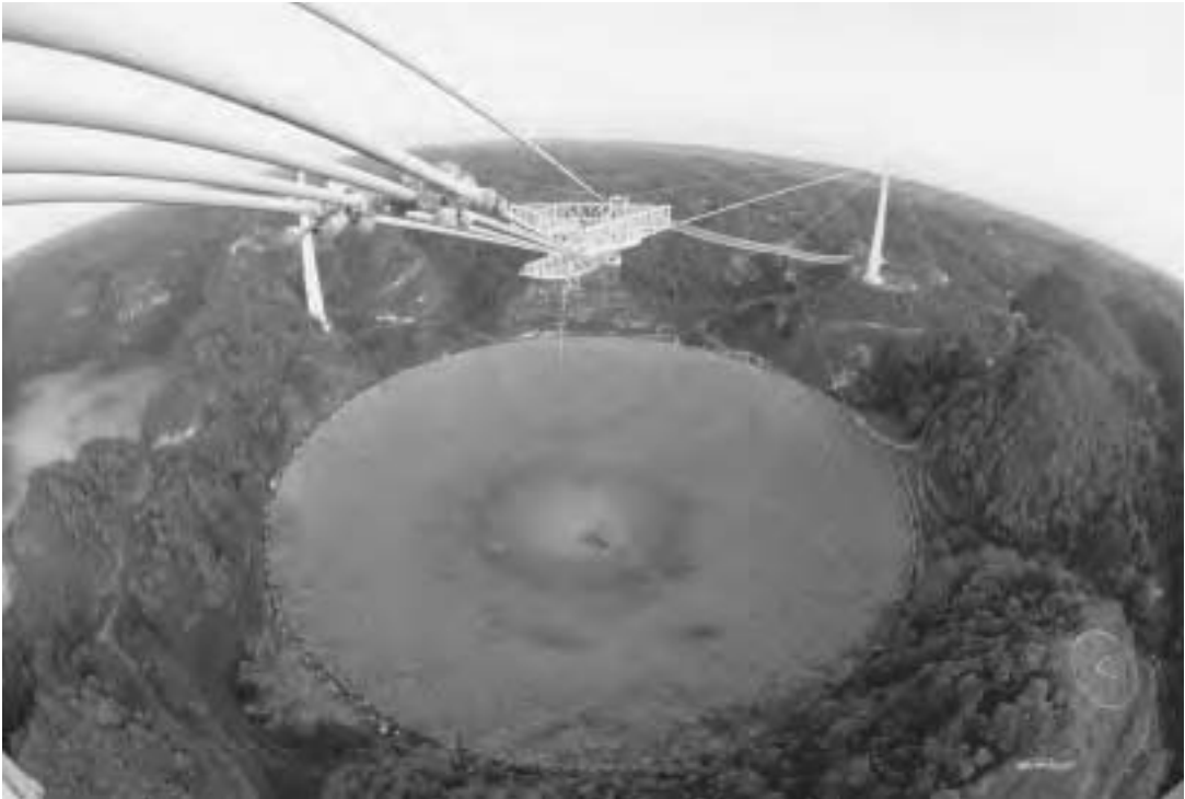
The 1,000-foot-wide dish of the Arecibo Radio Telescope as viewed from its cable-suspended receiver (Roger Ressmeyer/Corbis)
